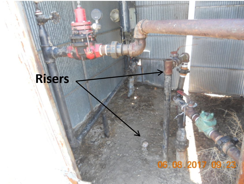
Photo 5. Unused 2" riser in shed. 2" riser open to atmosphere
