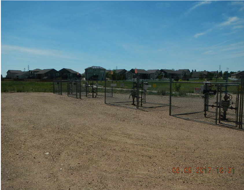
Wellheads and 2" risers
