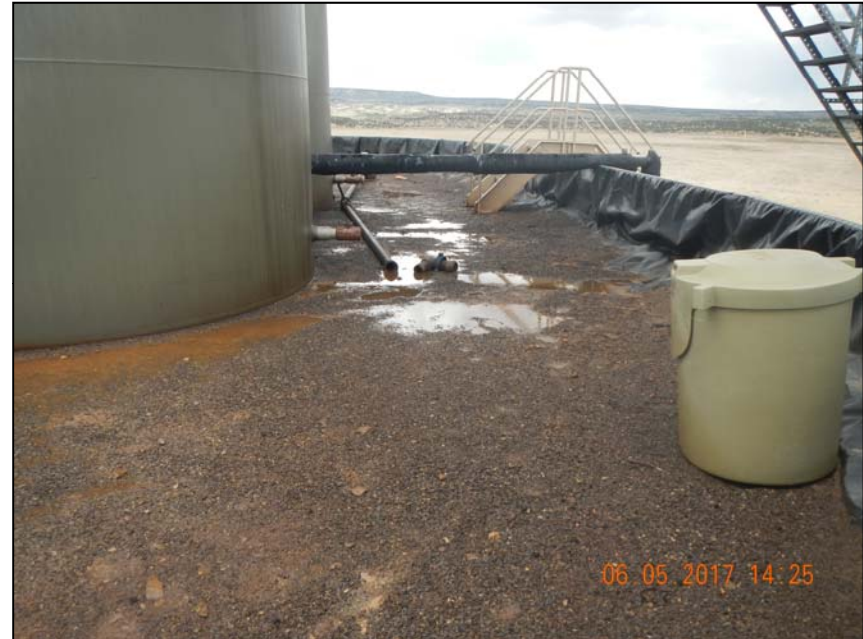
Photo 11. Produced water leak.
