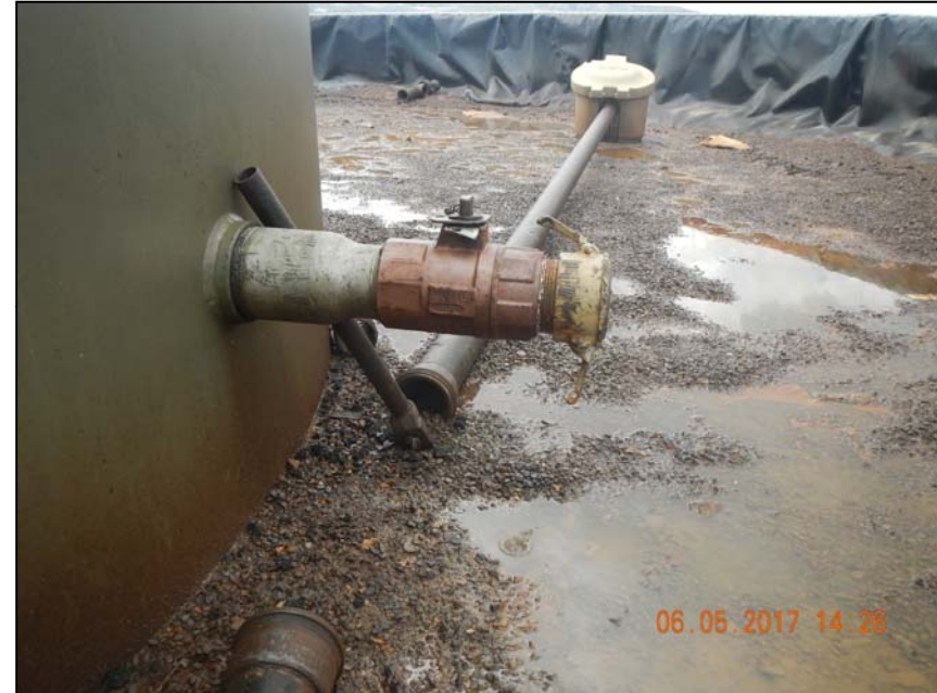
Photo 13. Source of spill and ongoing drip leak.
