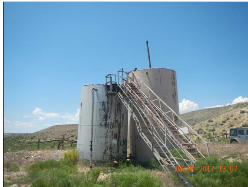
Photo 7. Unlabeled tanks. Open gauge hatch. No wildlife protection on exhaust.
