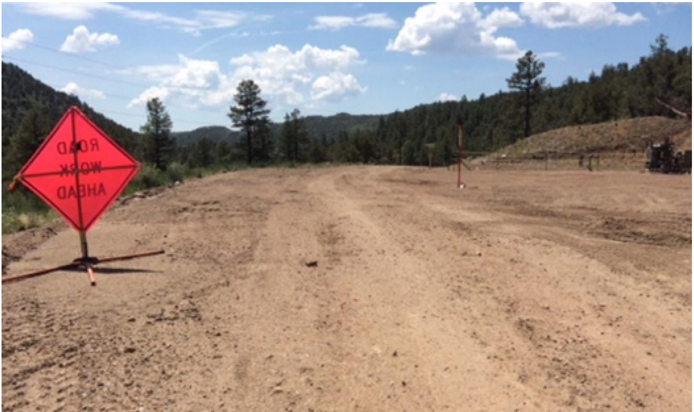
Photo 3: Facing south along the main road which goes through location. Pulled gravel back onto the driving surface.
