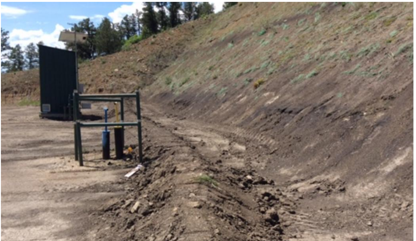
Photo 4: Facing southwest toward the cut slope of the location. The rills were raked out, the sediment accumulation was removed and a dirt berm was installed at the toe of the cut slope.
