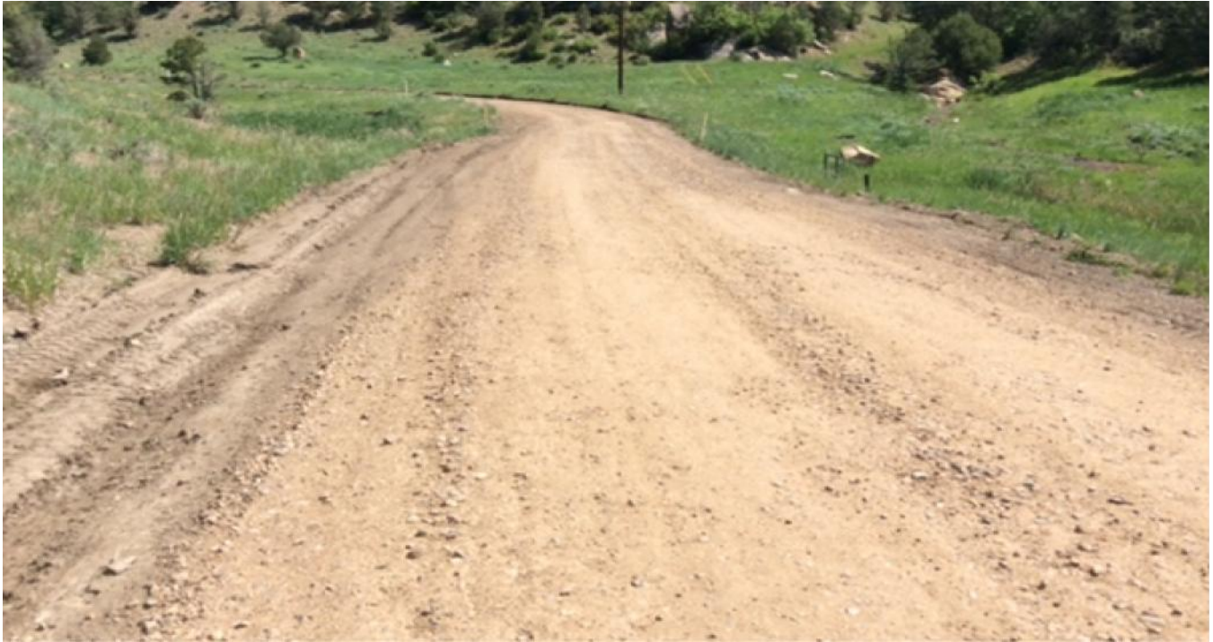
Photo 1: Facing northeast along the main access road. Installed gravel and crowned the driving surface to establish sheet flow.
