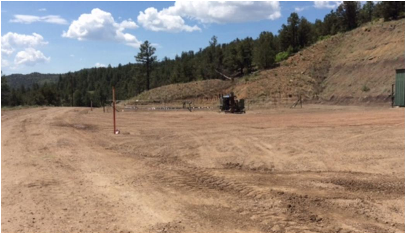
Photo 2: Pulled gravel back onto the driving surface.
