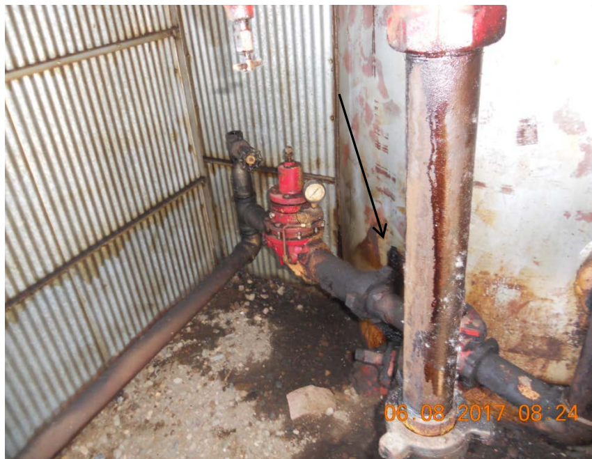
Photo 13. Second seep in treater wall
