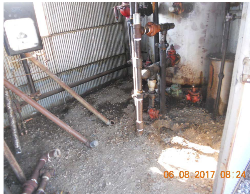
Photo 10. Stained soil in treater shed
