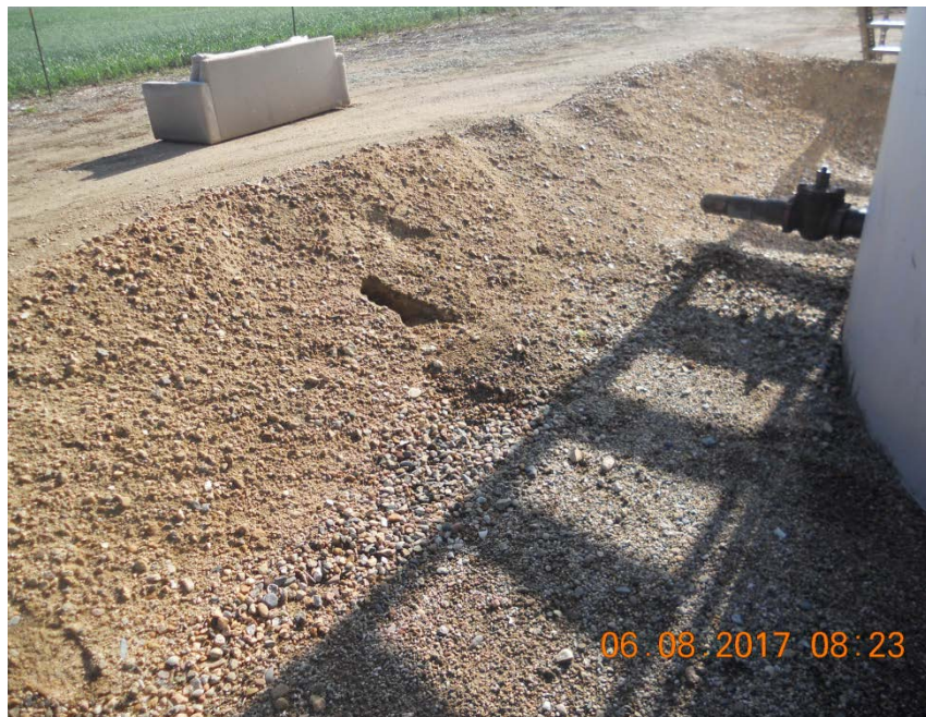
Photo 7. Animal burrow in berm.
