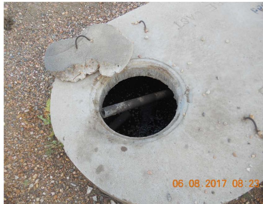
Photo 6. Open vault oily substance on water
