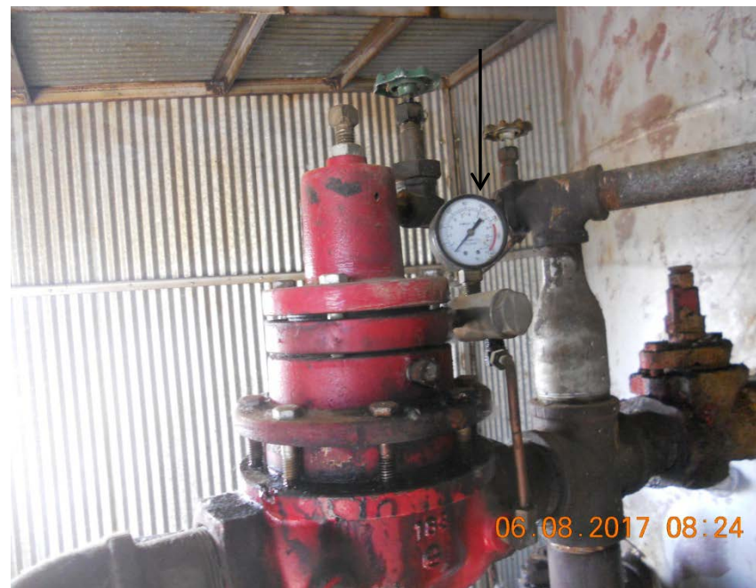
Photo 12. Gauge indicates no pressure on treater
