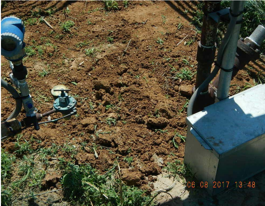
2" steel riser after process riser removal
