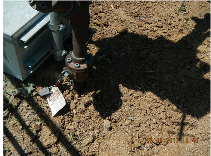
Stephens 7-15 2" steel riser after 1" process riser removal
