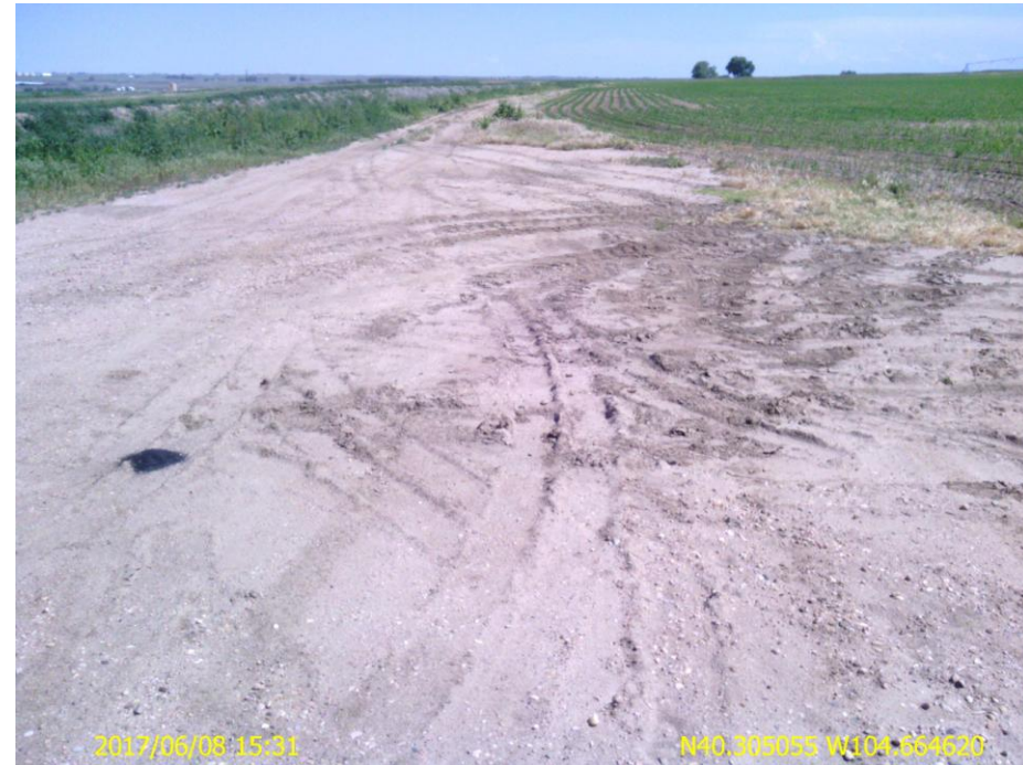
Photo 2: Photo taken from the battery location, facing south. Photo shows battery location and access road have not been reclaimed.
