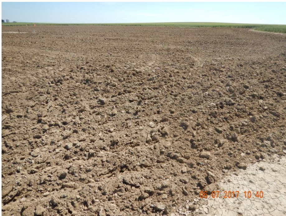
Photo 3: Photo taken from the south end of the location, facing northeast. Photo shows location has had surface roughening implemented. Surface roughening is a temporary BMP that should be used in conjunction with other BMPs. Photo also shows no perimeter BMP controls have been installed.
