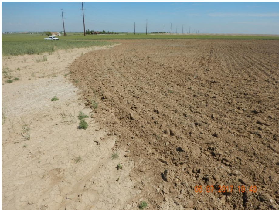
Photo 1: Photo taken from the south end of the location, facing northwest. Photo shows location has had surface roughening implemented. Surface roughening is a temporary BMP that should be used in conjunction with other BMPs. Photo also shows no perimeter BMP controls have been installed.
