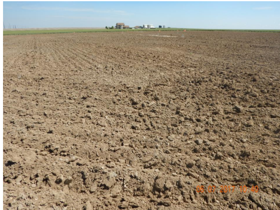
Photo 2: Photo taken from the south end of the location, facing north. Photo shows location has had surface roughening implemented. Surface roughening is a temporary BMP that should be used in conjunction with other BMPs. Photo also shows no perimeter BMP controls have been installed.
