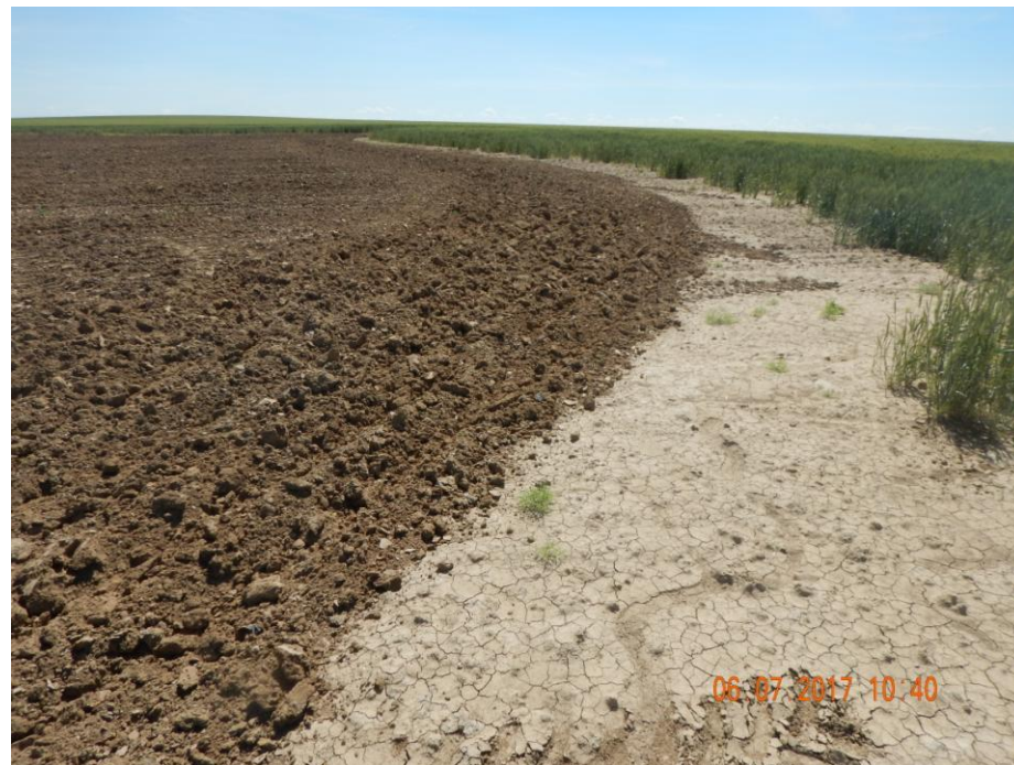
Photo 4: Photo taken from the south end of the location, facing east. Photo shows location has had surface roughening implemented. Surface roughening is a temporary BMP that should be used in conjunction with other BMPs. Photo also shows no perimeter BMP controls have been installed.
