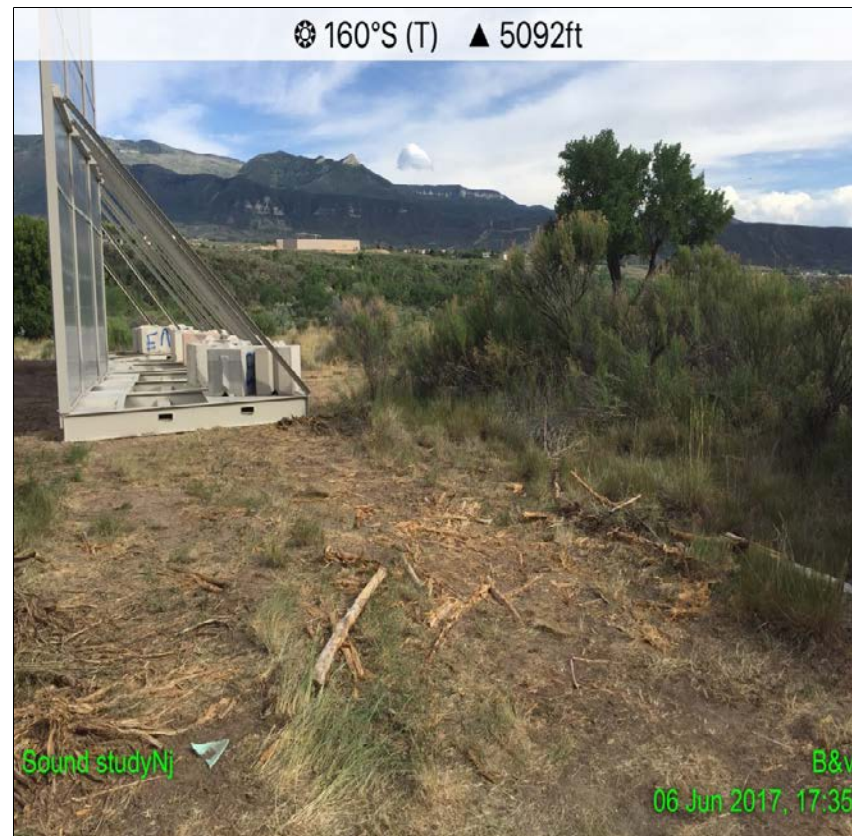
Vegetation and soil disturbance with no Storm water BMP in place.
