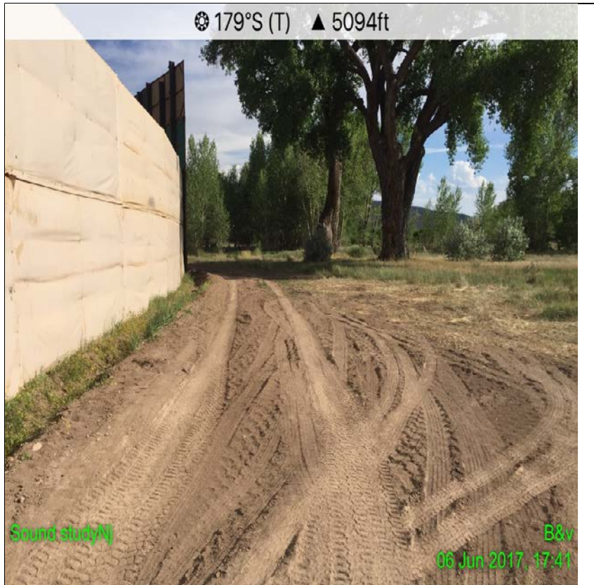
Access Road way with no Storm Water BMP in place
