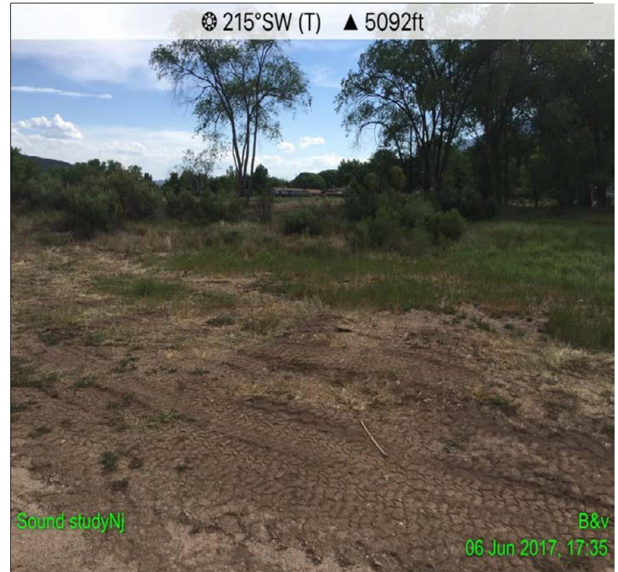
Soil and vegetation disturbance with no Storm water BMP in place.
