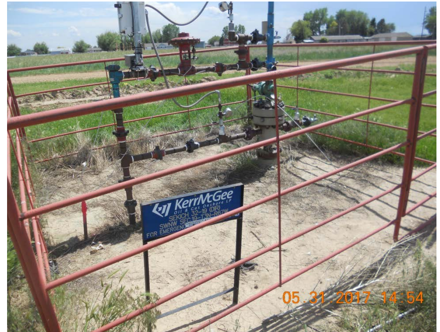
Sekich 32-19 2" flowline in use 1" riser to be abandoned
