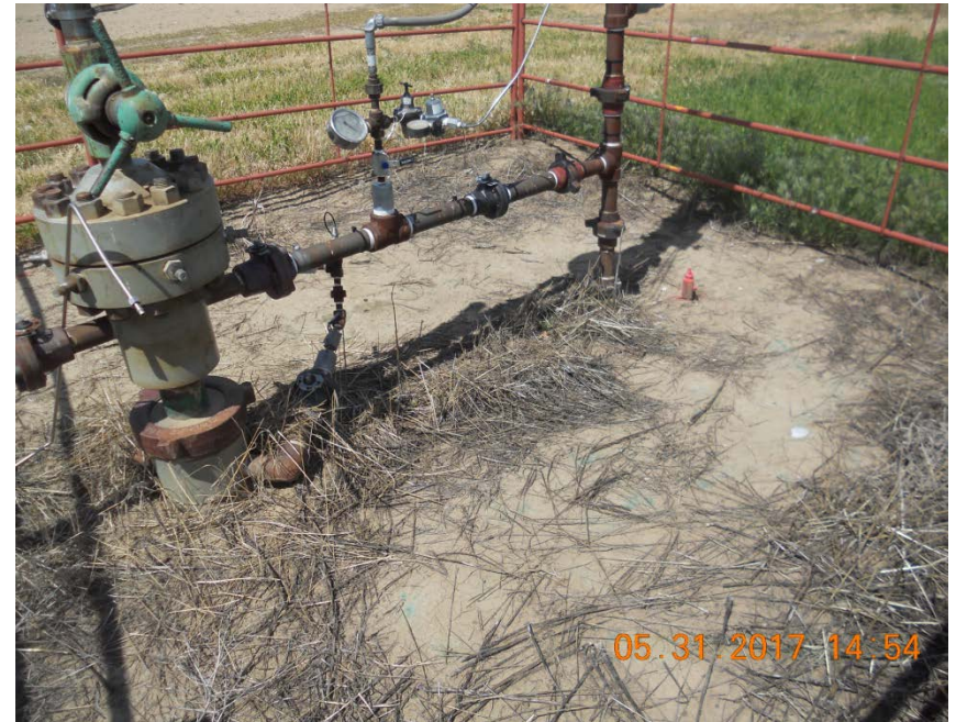
Sekich 22-19 2" flowline in use 1" riser to be abandoned
