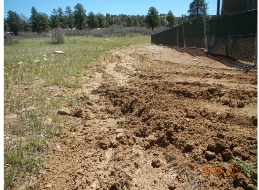
Photo 4: View of northern diversion facing eastward, damaged with deep ruts and disturbed soil. Diversion needs repair and stormwater controls.
