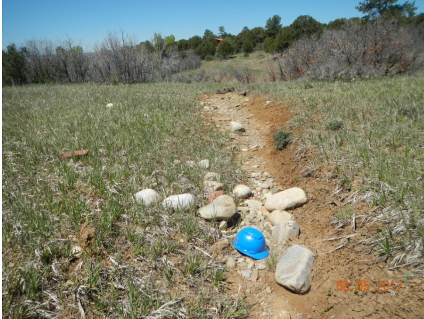
Photo 3: View of erosion occurring within the northern portion of the project area facing westward. Stormwater controls need to be installed to de-energize flows.
