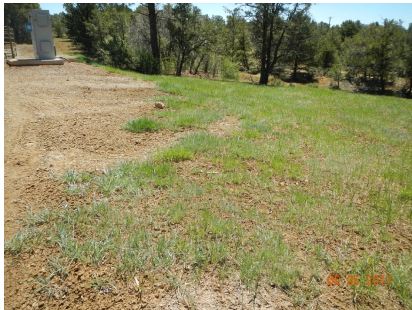
Photo 4: View of area along the southeastern edge of the well pad where concentrated stormwater flows off of the working area and is starting to cause erosion.
