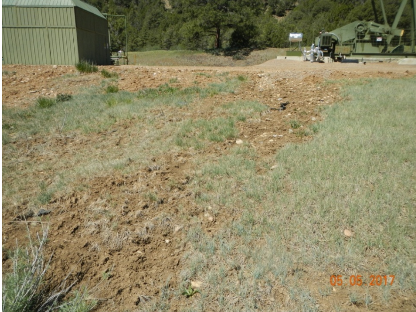
Photo 3: View of area along the eastern edge of the working area where concentrated stormwater flows off of the well pad and is eroding the interim reclamation area.
