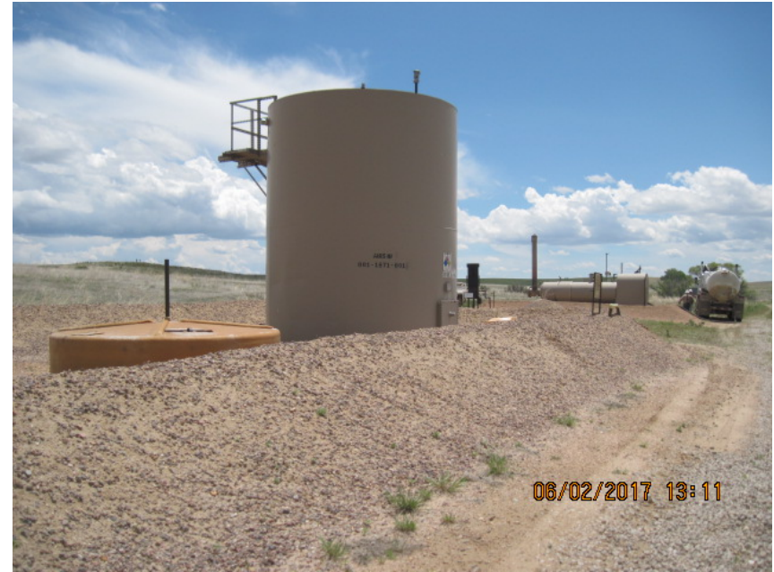
TANK BATTERY AND EQUIPMENT
