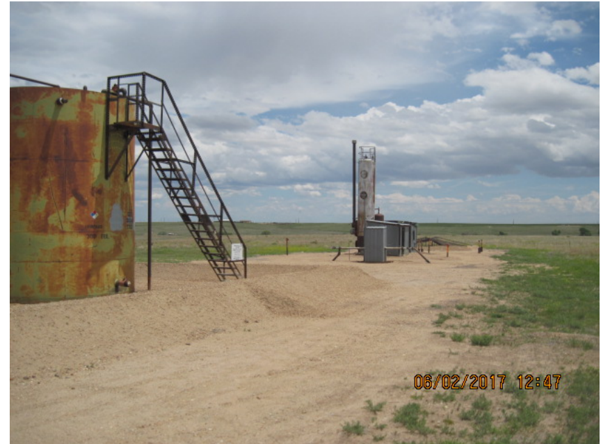
TANK BATTERY AND EQUIPMENT
