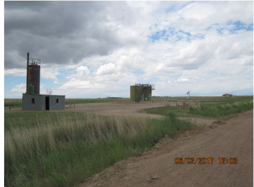
TANK BATTERY AND EQUIPMENT
