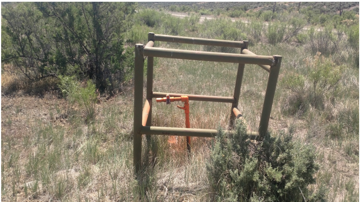
Riser #2: Blackhills operated gathering line drip line connected to 6" active gathering line.
