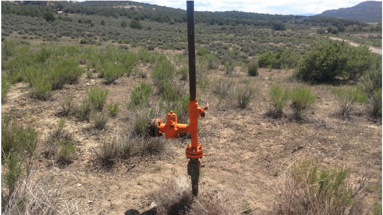
Riser #1: Blackhills operated gathering line riser. Connected to an active 6" gathering line. Formally connected to a meter run (downstream of meter run).
