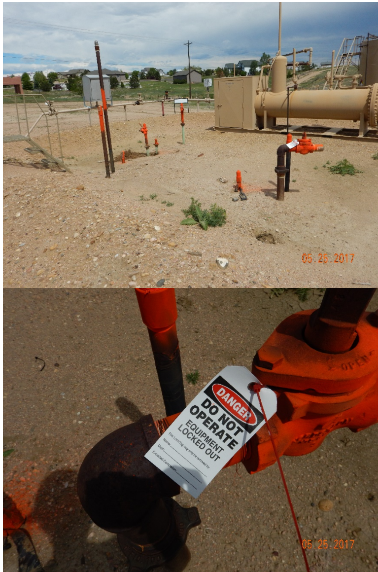
Photos 5 & 6 - Abandoned flowline risers at former TTOC battery location have been tagged and painted by COGCC, per 2017 Flowline NTO.
