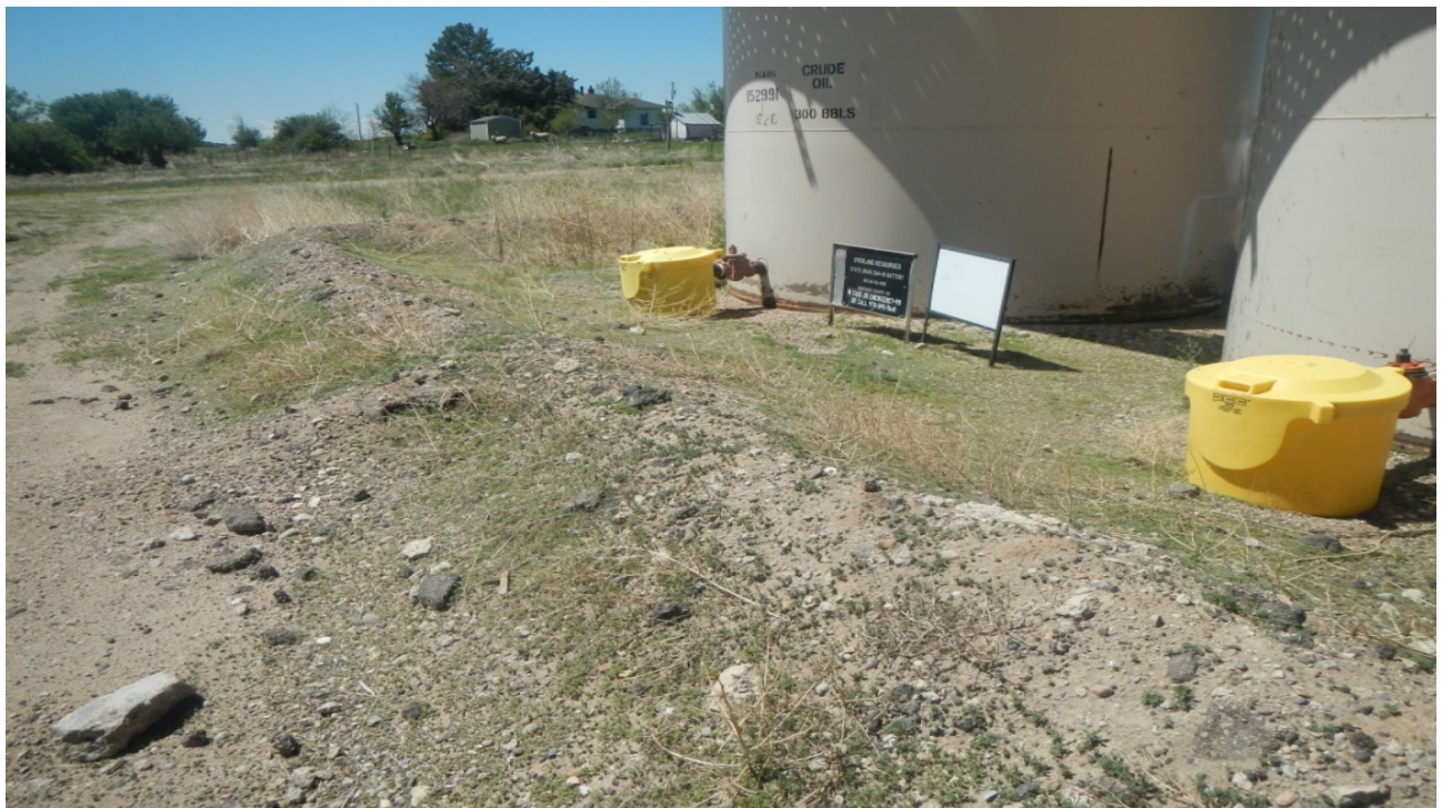
photo 2: There is weeds and vegetation growing inside the berm and around the equipment.
