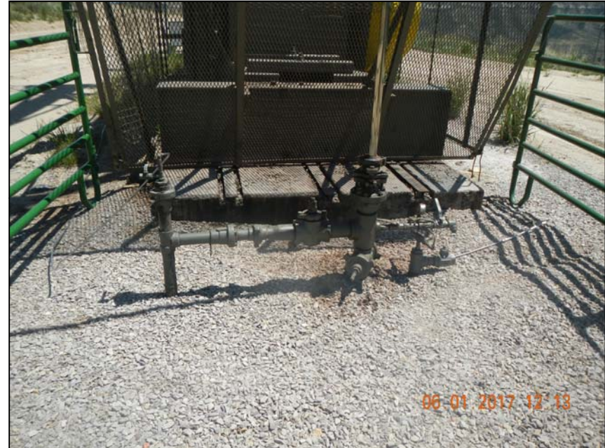
Photo 2. 1 – 2” and 1 – 3” steel riser at wellhead.
