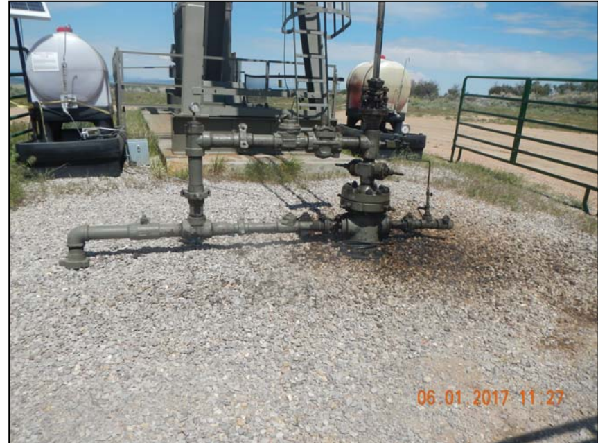
Photo 2. 1 – 2" steel riser at wellhead. Stained soil at wellhead.
