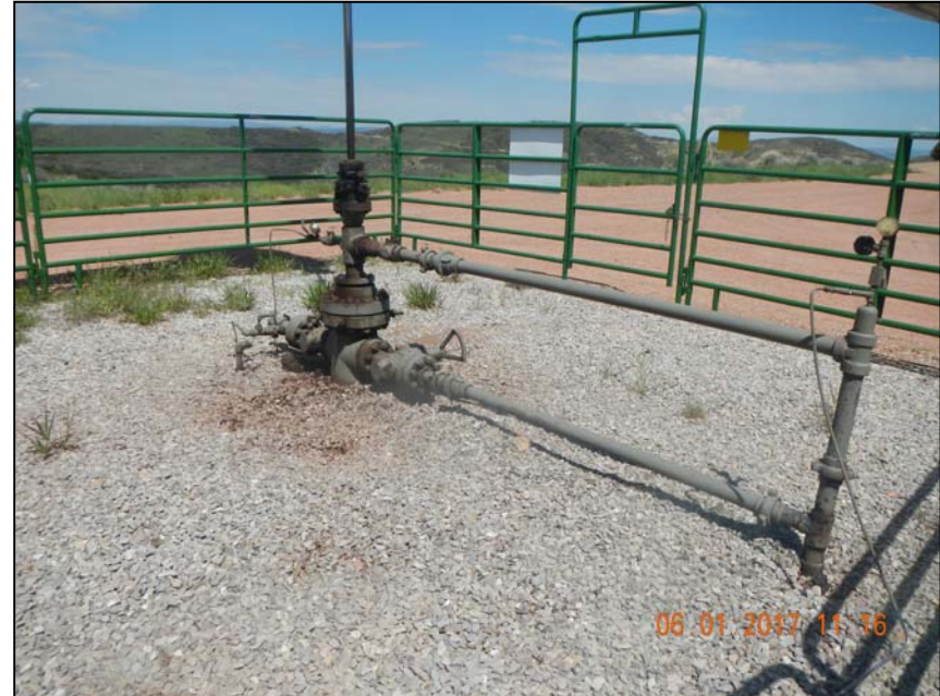
Photo 2. 1 – 2” and 1 – 1” steel riser at wellhead.
