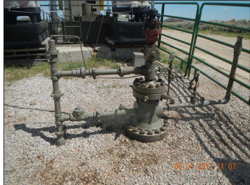
Photo 2. 1 – 2" steel riser at wellhead.
