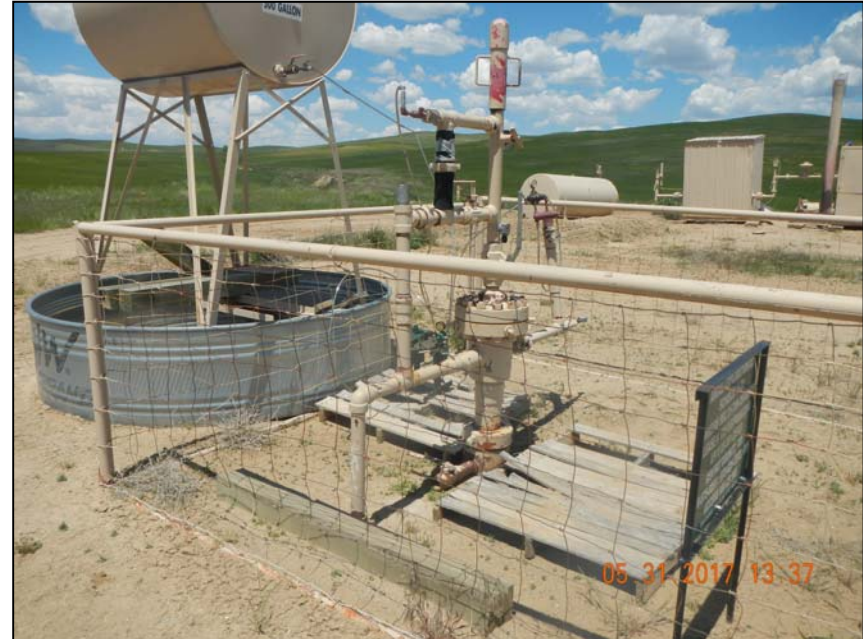
Photo 2. 1 – 2" steel riser at wellhead.
