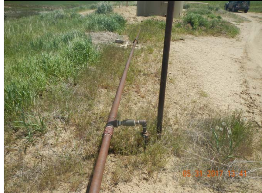
Photo 6. Steel flowline from separator to tank with 1 – 1" steel riser at midway point.
