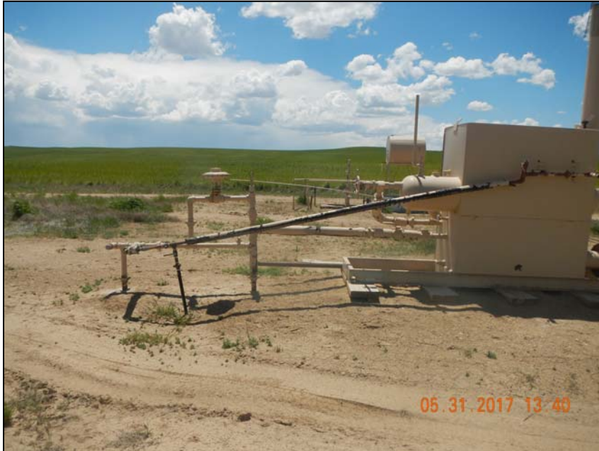
Photo 5. 2 – 2" and 1 – 1" steel risers at separator.
