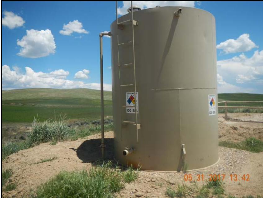
Photo 7. 1 – 2" steel riser at tank.
