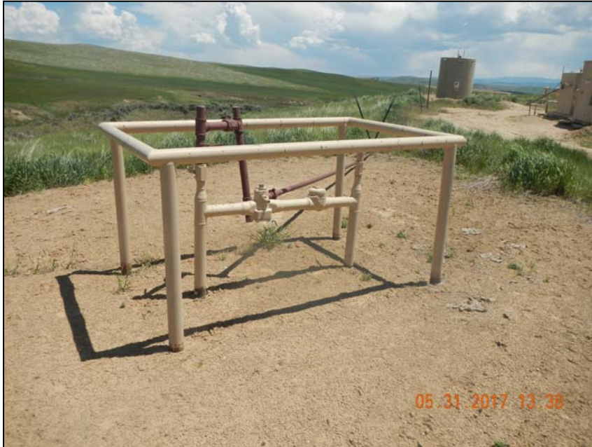
Photo 3. Riser cluster with 2 – 2” and 1 – 1” steel risers at 40.60605, -107.53705
