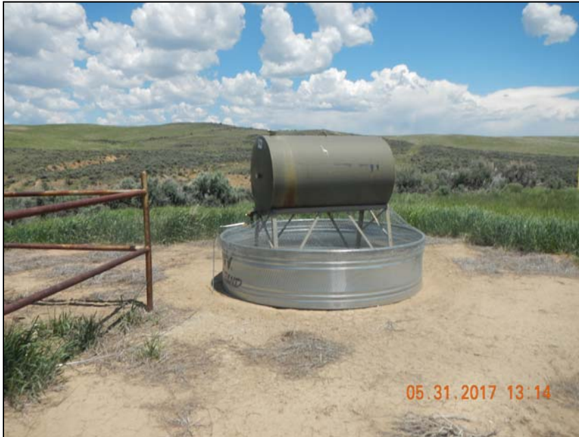
Photo 3. Unlabeled container at wellhead.
