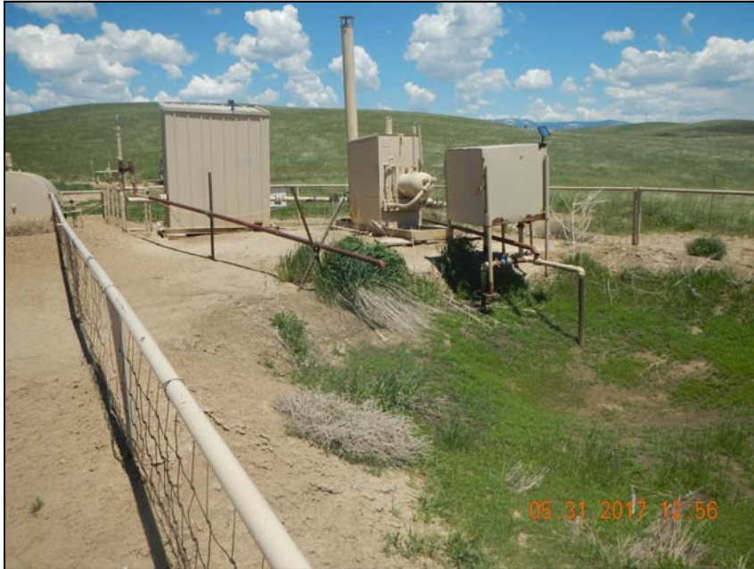
Photo 3. Pit with separator and meter run and risers.
