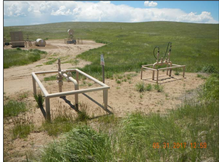
Photo 4. Riser cluster with 4 – 2” insulated steel risers at 40.61253, -107.52946
