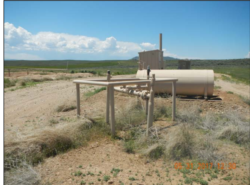
Photo 5. Riser cluster with 3 – 2” insulated risers at 40.61391, -107.54092
