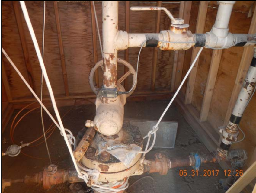
Photo 2. Wellhead with 1 – 2” riser on right.
