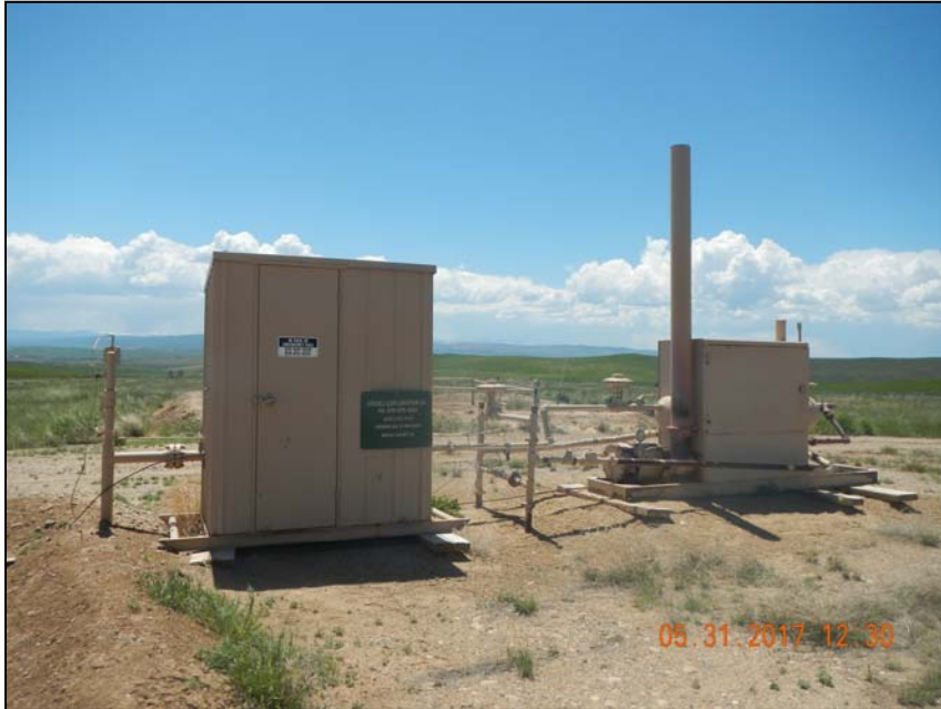
Photo 4. Meter run with 1 – 2” steel riser and separator with 2 -2” steel risers.
