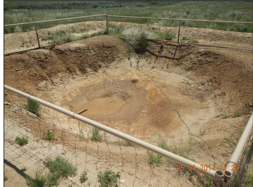
Photo 3. Pit with 2” steel flowline entering from separator.
