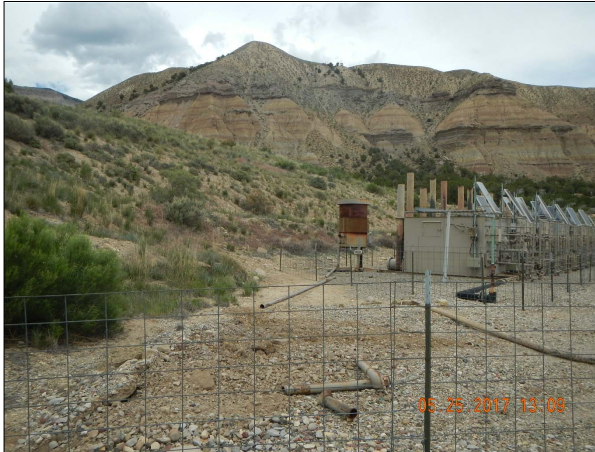
Flow line from tanks to combustor is disconnected and ready for removal .
