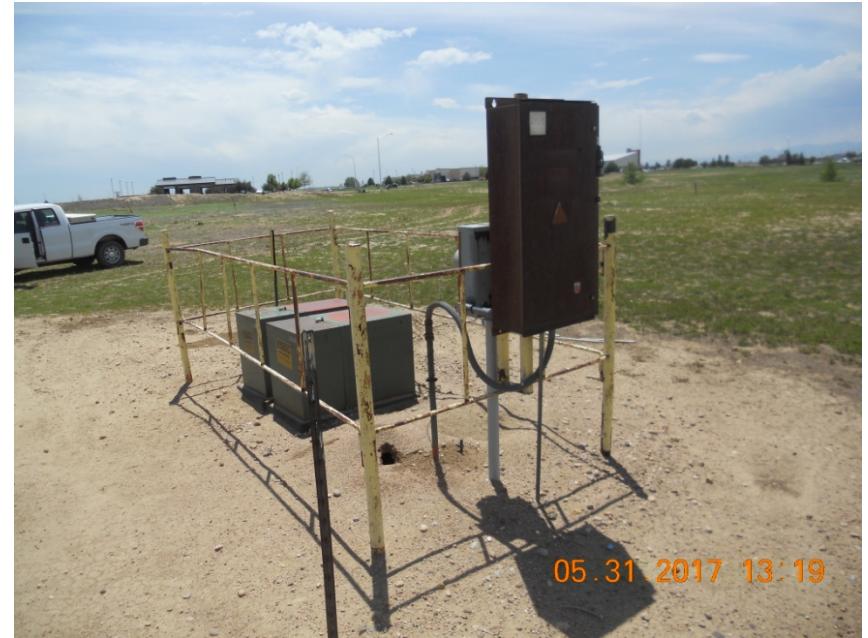
Power box and transformers west of pumpjack
