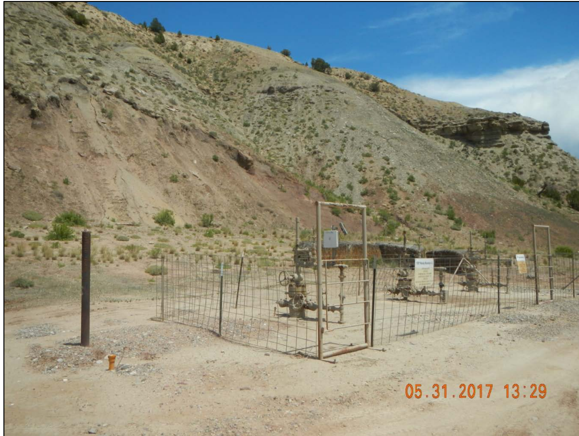
Unused riser painted orange at plugged and abandoned well GM 513-1
