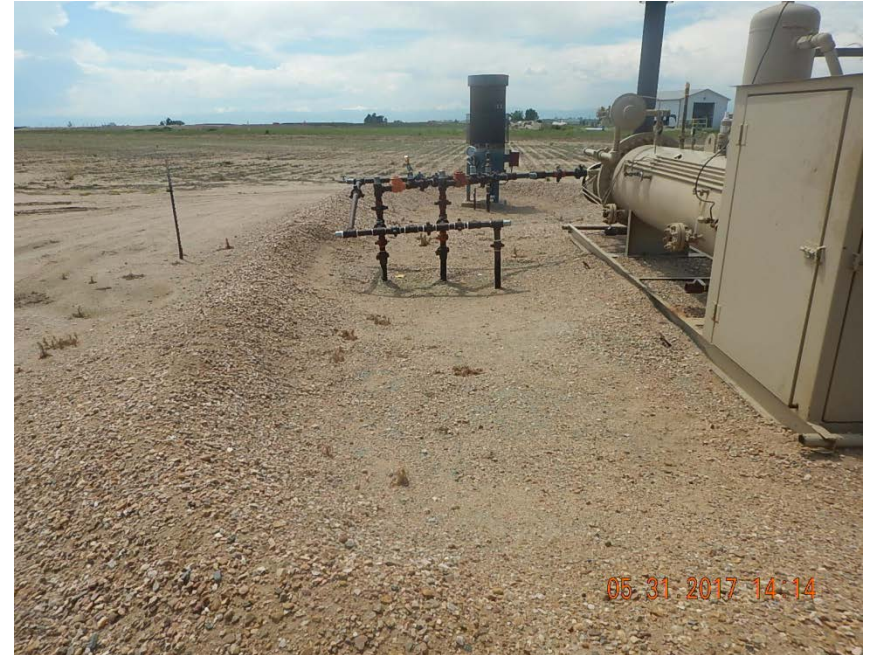
Photo 4: Risers at separator
