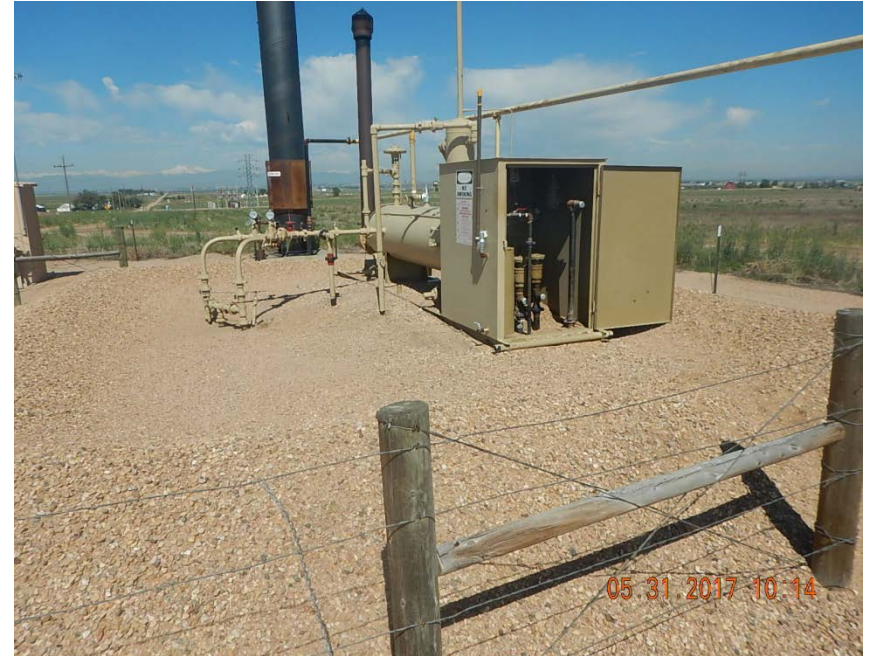
Photo 4: Risers at separator
