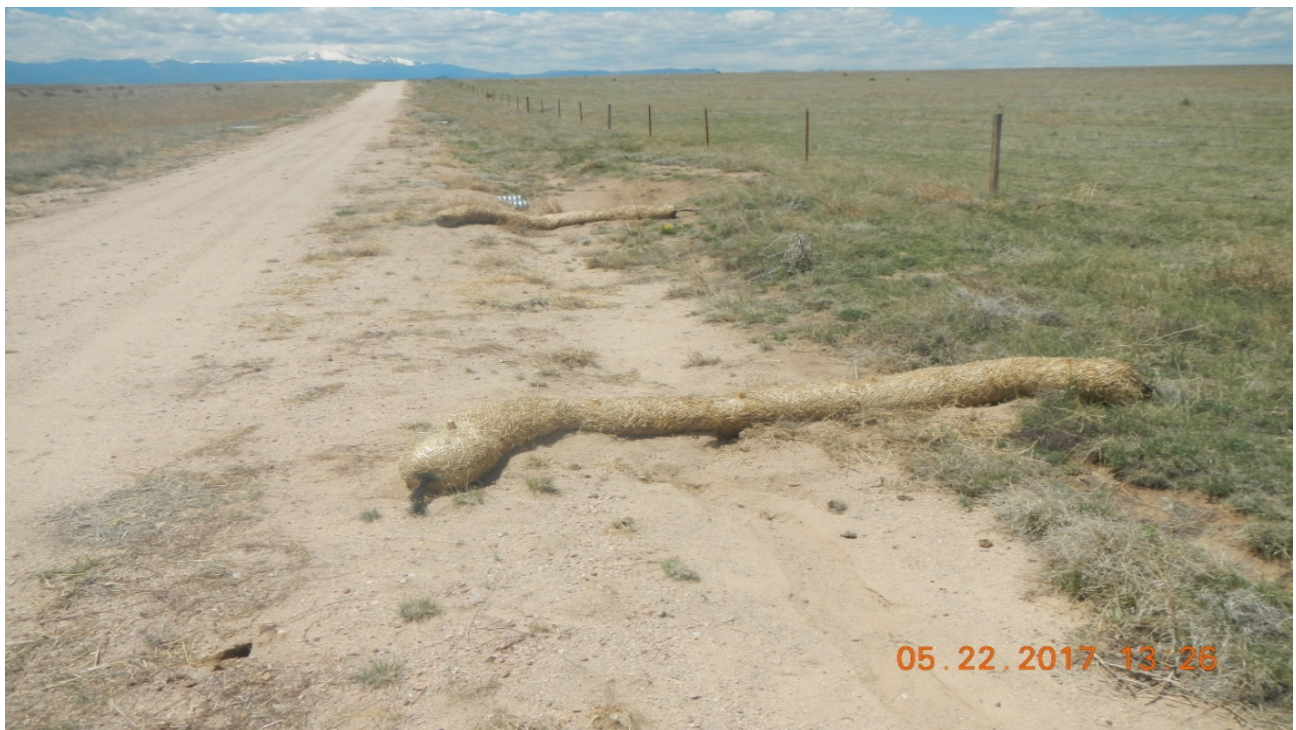
photo 8: Straw wattles are installed along the access road near this culvert.
