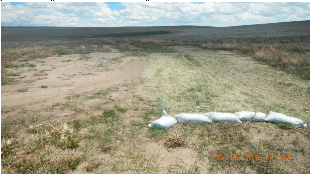
photo 18: Facing south at the location. It appears that the area of the right side of the photo was seeded and a straw blanket was installed. It does not appear the area at the left side was seeded.
