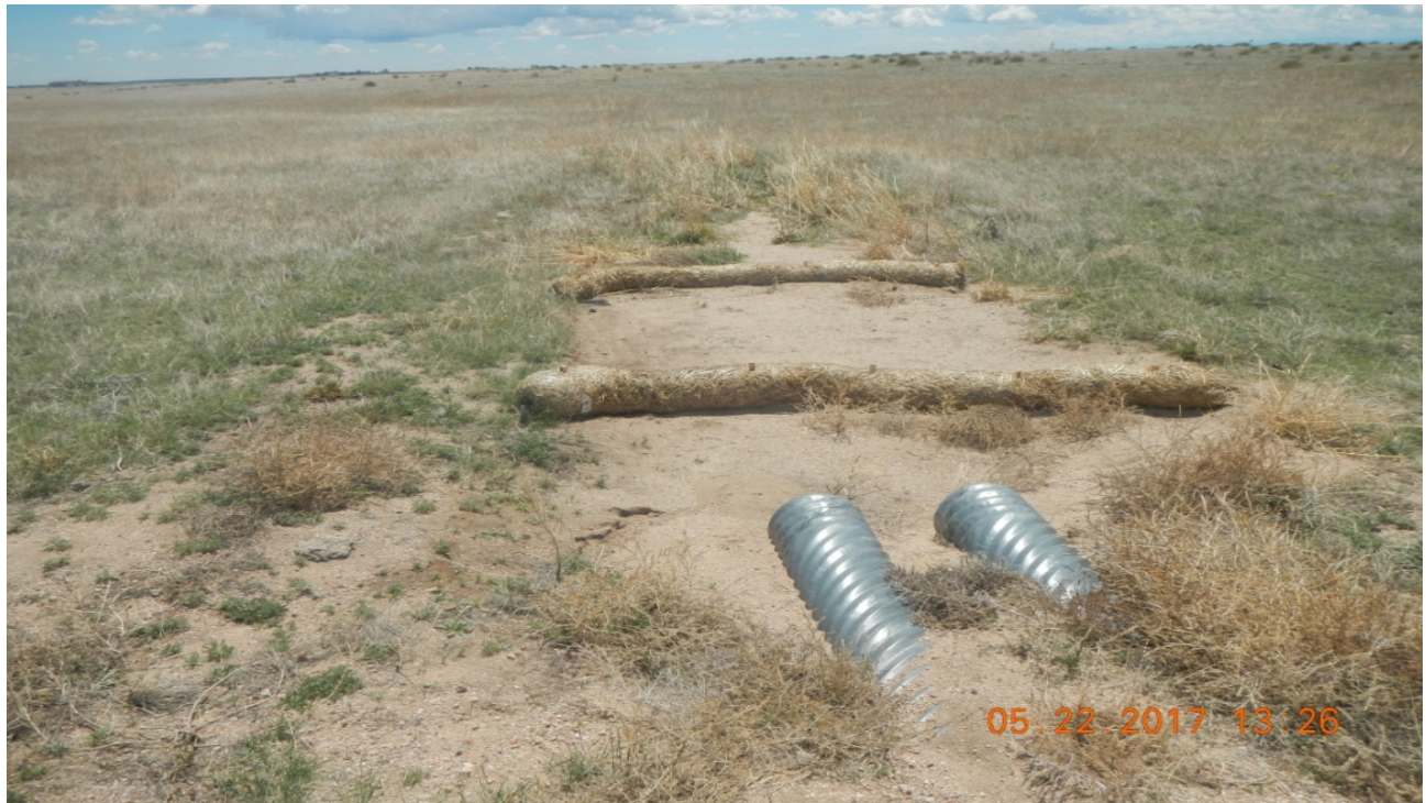
photo 9: The outlet of the culvert along the access road. The sediment has not been removed which will restrict water flow. Straw wattles were installed.
