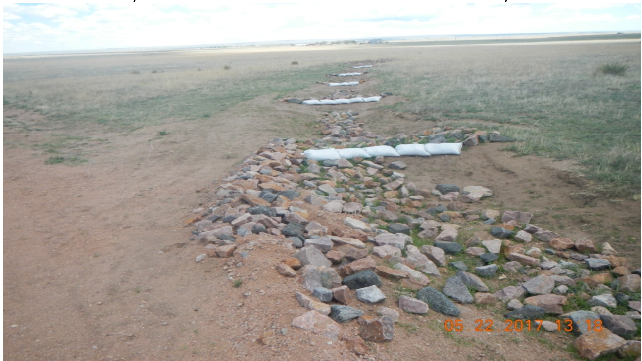
photo 4: The erosion channel directed out toward the pasture has rock rip/rap and sandbags installed.
