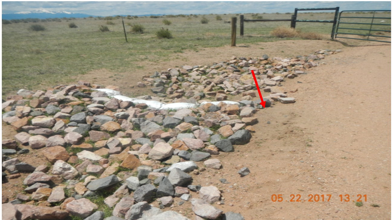
photo 3: There are rock rip/rap check dams with sandbags however they don't appear to be constructed correctly. Stormwater could flow around the low area as shown by the arrow.
