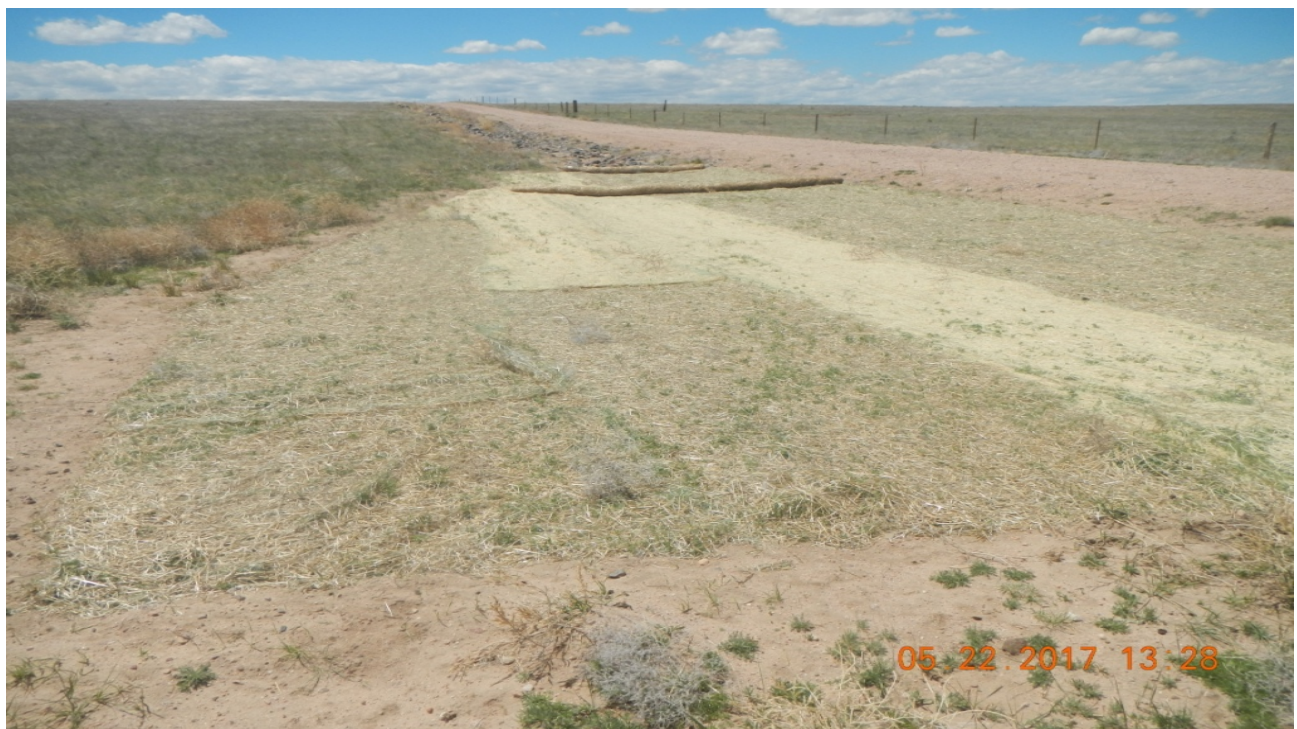
photo 10: Facing northwest along the side of the access road. Erosion straw blanket was installed and there appears to be vegetation beginning to establish.
