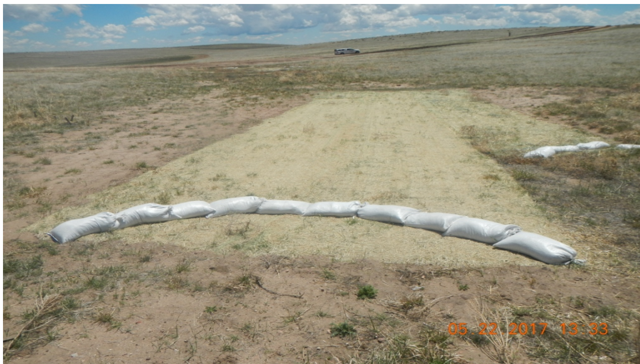
photo 13: Straw blanket and sand bags are installed in this area.
