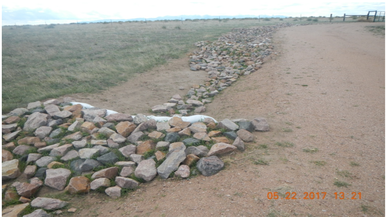
photo 2: Facing west along the access road. Rock rip/rap has been placed along the road where erosion channel was documented in the previous inspection.
