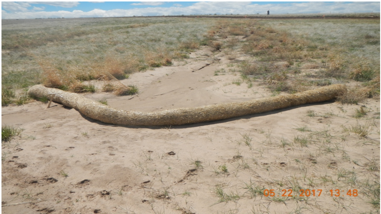
photo 22: There are signs that stormwater is eroding underneath the straw wattle which was not properly installed.
