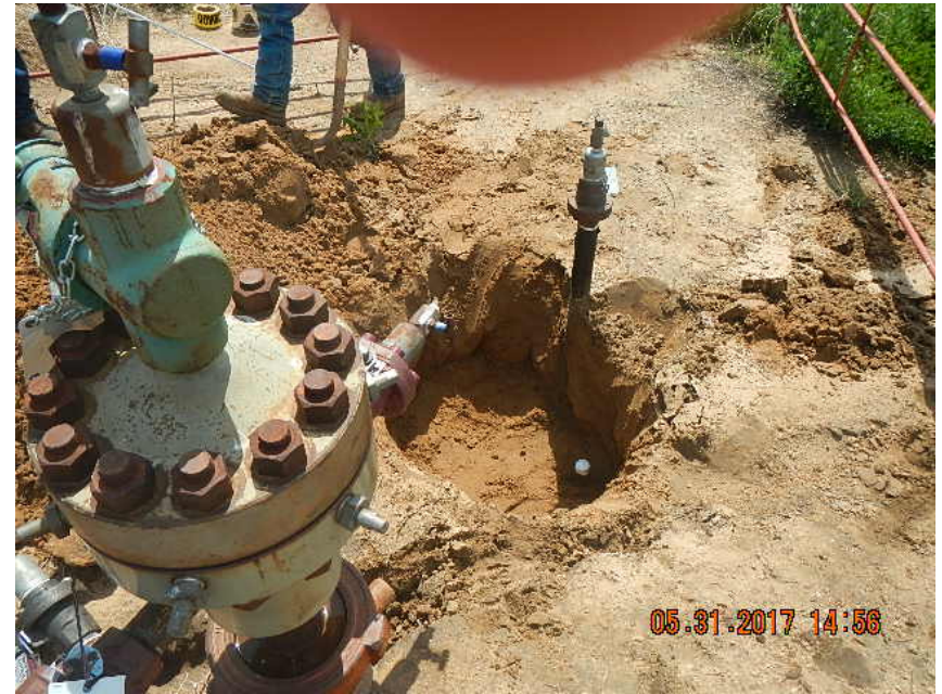
1" STEEL RISER ABONDONMENT PER NTO
