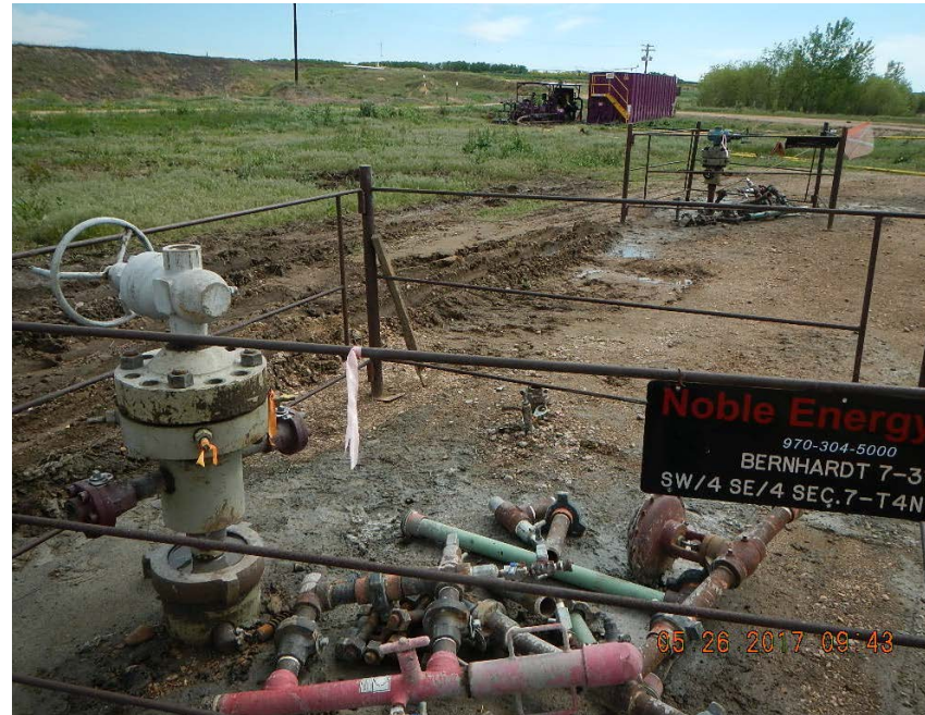
Wellhead and flow lines
