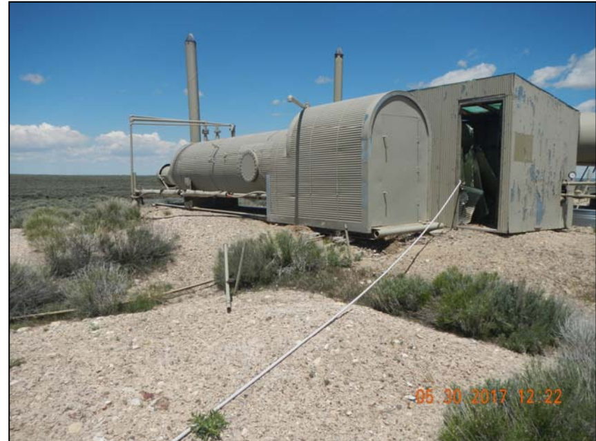
Photo 5. Risers at separator with poly flowline in foreground.
