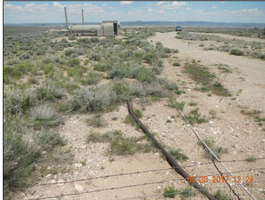
Photo 8. Flowlines from tank battery to separator and pit.
