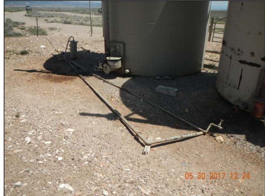
Photo 7. Risers at tank battery.
