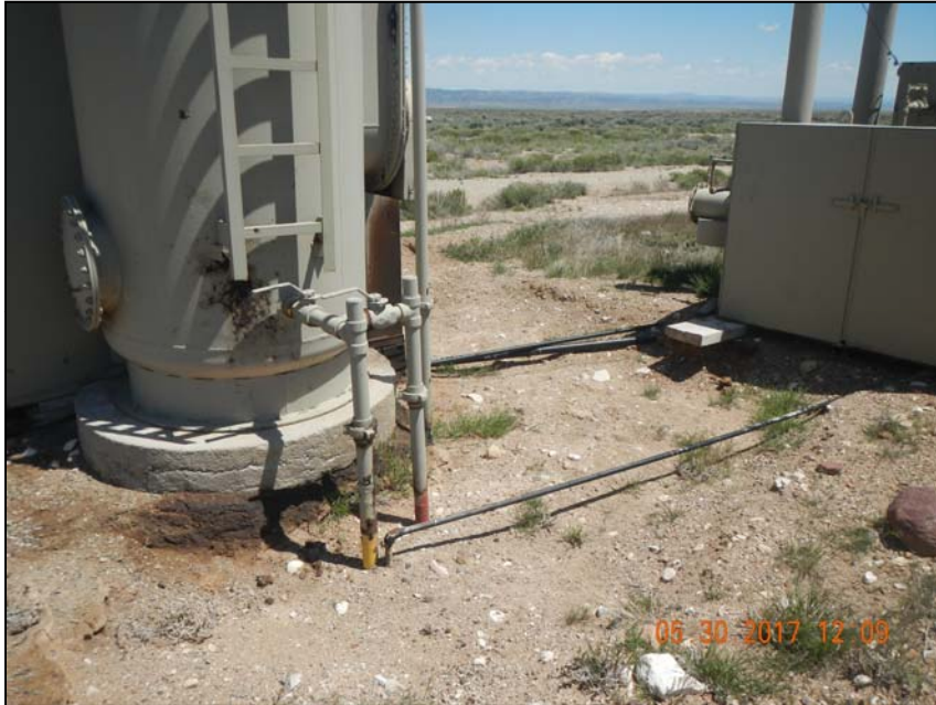
Photo 8. Risers and flowlines at vertical and middle horizontal separators.
