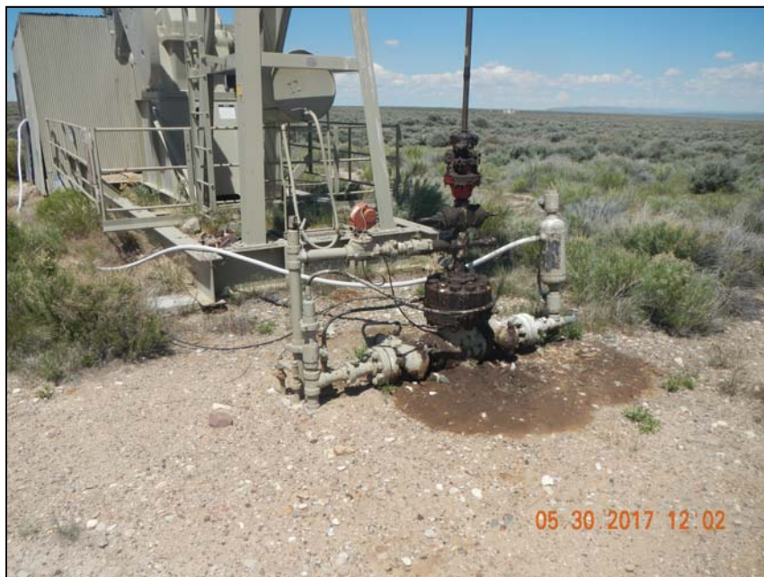
Photo 2. Risers at wellhead. Stained soil at wellhead.
