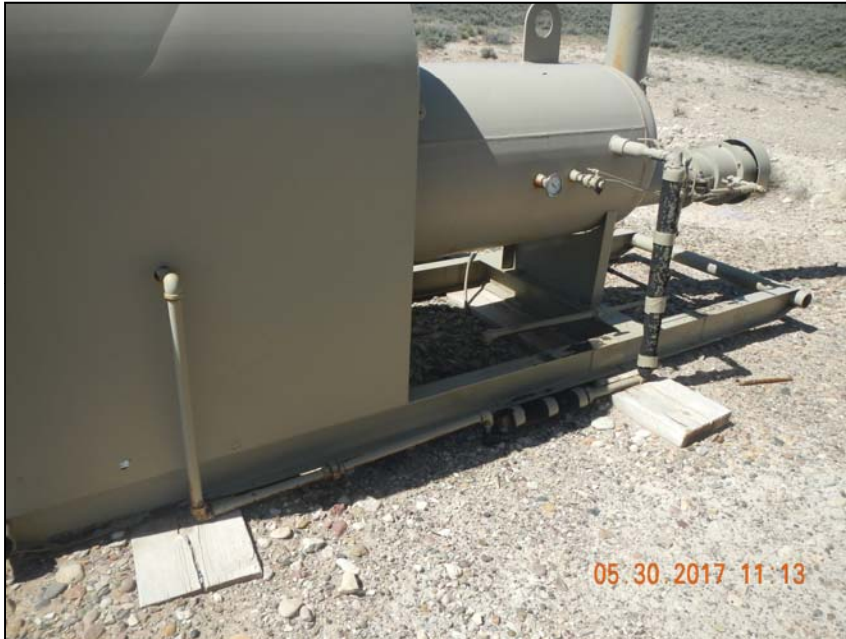
Photo 8. 3 – 1” steel risers at horizontal separator.
