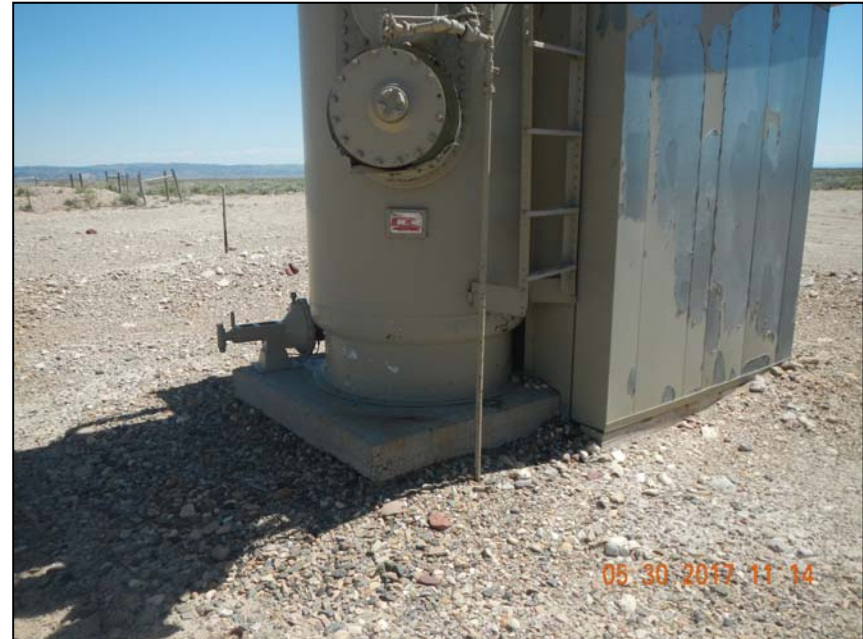
Photo 9. 5 -2” steel risers and 2 – 1” steel risers at vertical separator.
