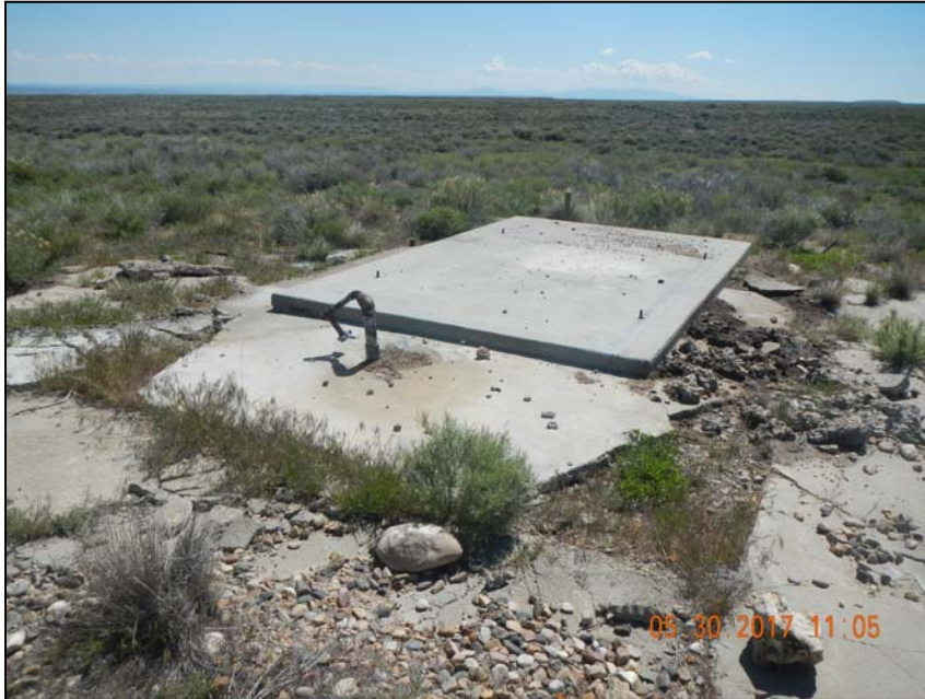
Photo 2. Concrete base at entrance with 4 – 2" steel risers not in use.
