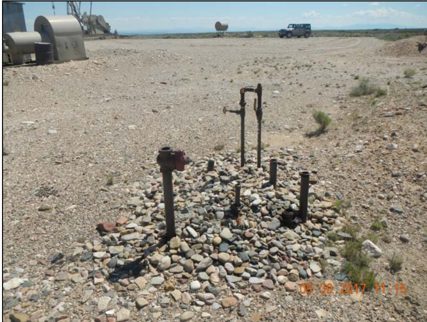
Photo 10. 5 – 2” steel risers and 3 – 1” steel risers not in use.
