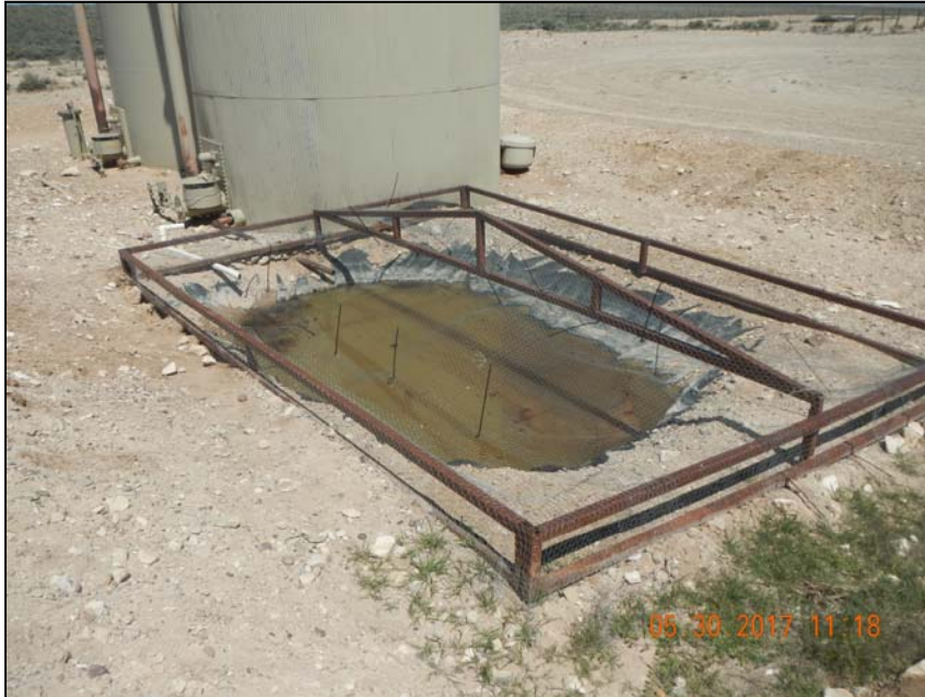
Photo 12. Pit in tank berm with sheen and oil and two flowlines entering from tank battery.
