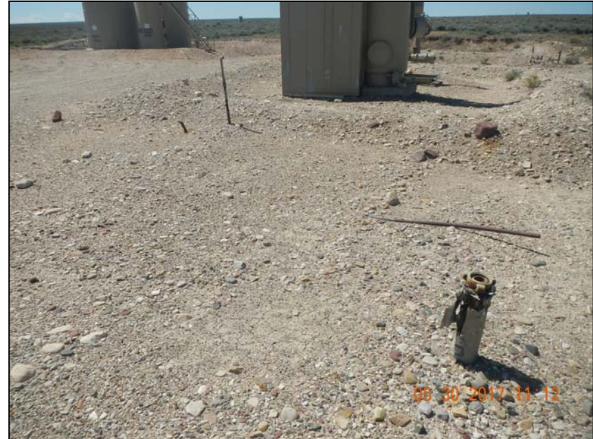
Photo 7. 1 – 2” and 1 -1” steel riser not in use.
