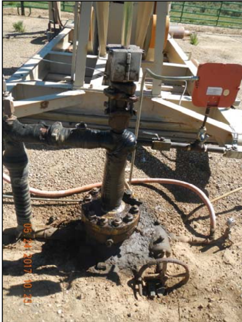
Photo 2. Stained soil at wellhead.
