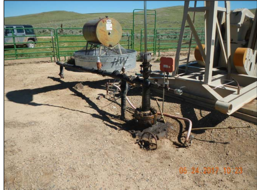
Photo 3. Wellhead assembly showing 1 -2" insulated riser, 1 -1" poly line, methanol lines.
