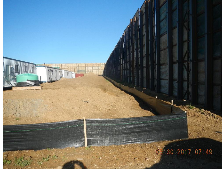
Photo 2 Silt fence and ditch from east
