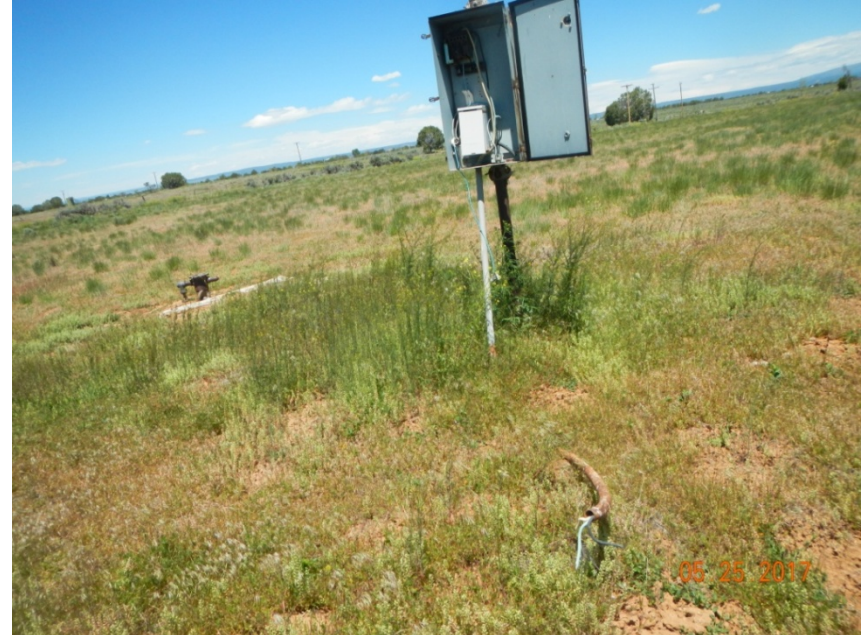
Photo 4: Another view of the electrical box and exposed wires (in foreground).
