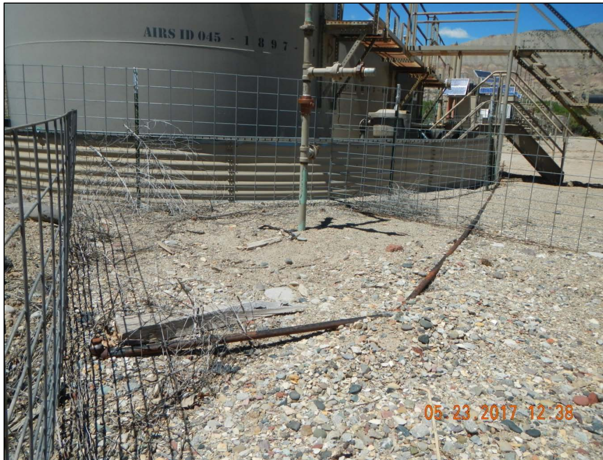
Gas supply line from separator for a removed combustor.
