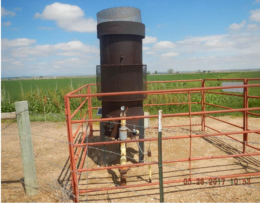
Photo 5 Emission control burner
