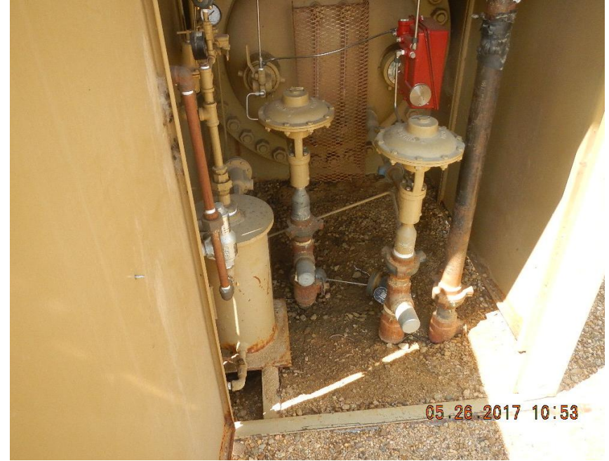
Photo 4 Flow lines within separator doghouse
