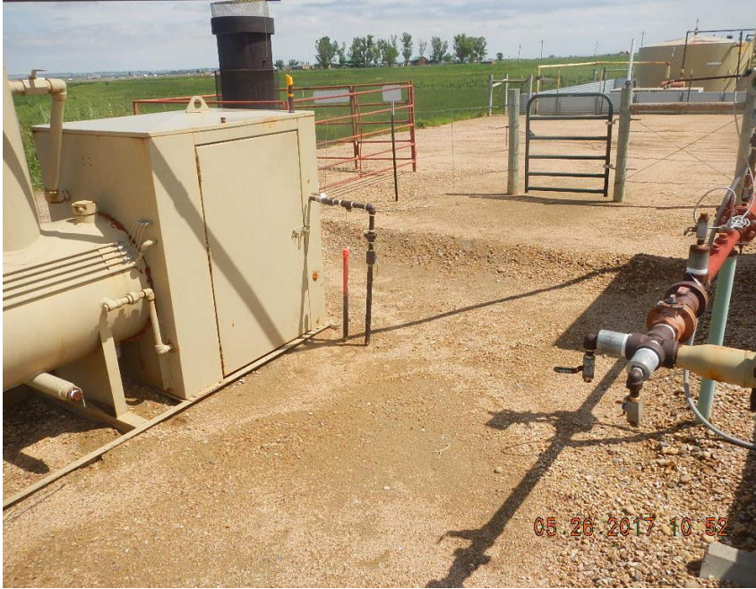
Photo 3 Flow lines at separator outlet
