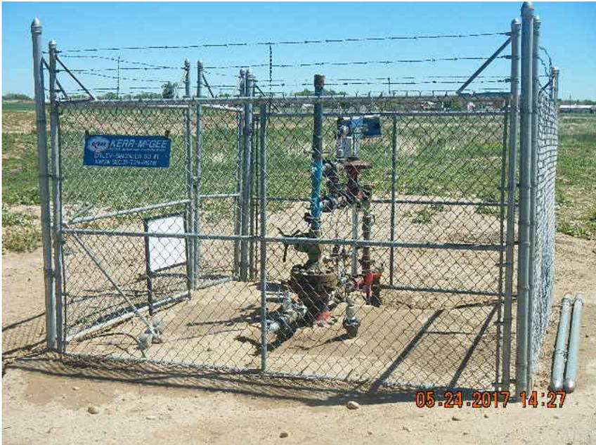
**Well head taken from North riser marked and capped per NTO**
