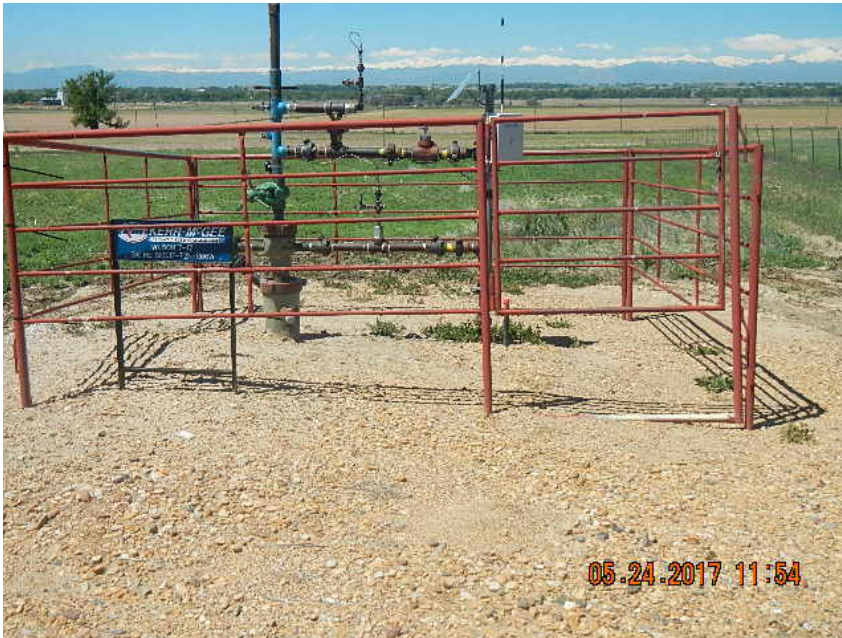
Well head taken from East riser marked and capped
