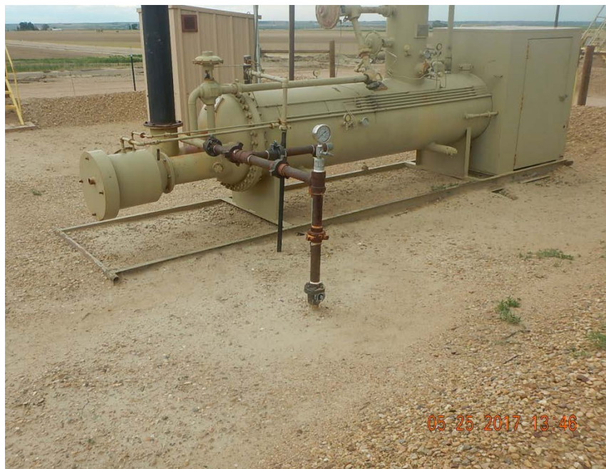
Photo 5: Risers at separator
