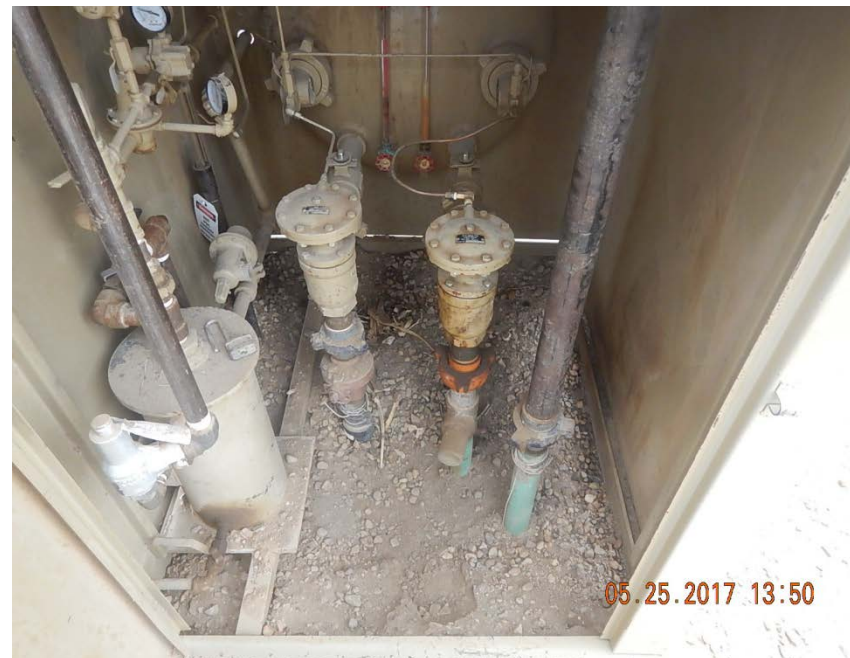
Photo 2: Risers in separator house
