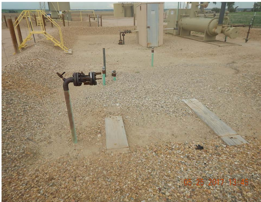
Photo 7: Risers from removed separator.
