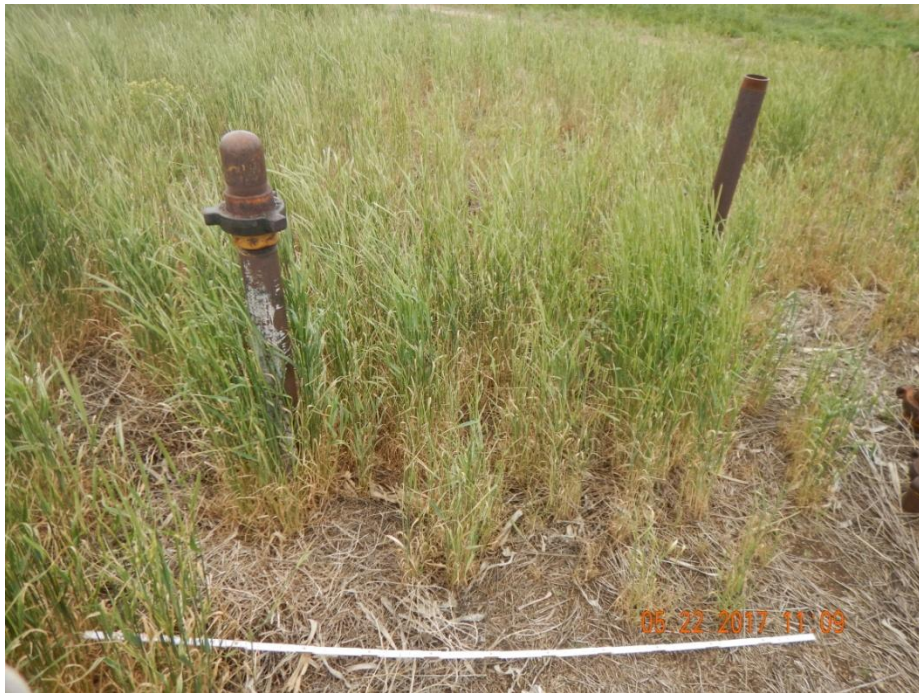
Photo 23: Photo of “~4 inch multi line w/ ~4 inch risers x2”
