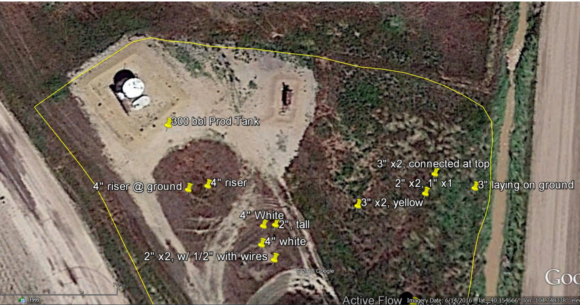
Photo 3: 2016 Aerial image. Photo shows location of all pipe risers inspector was able to locate remaining on the northern half of the location .
