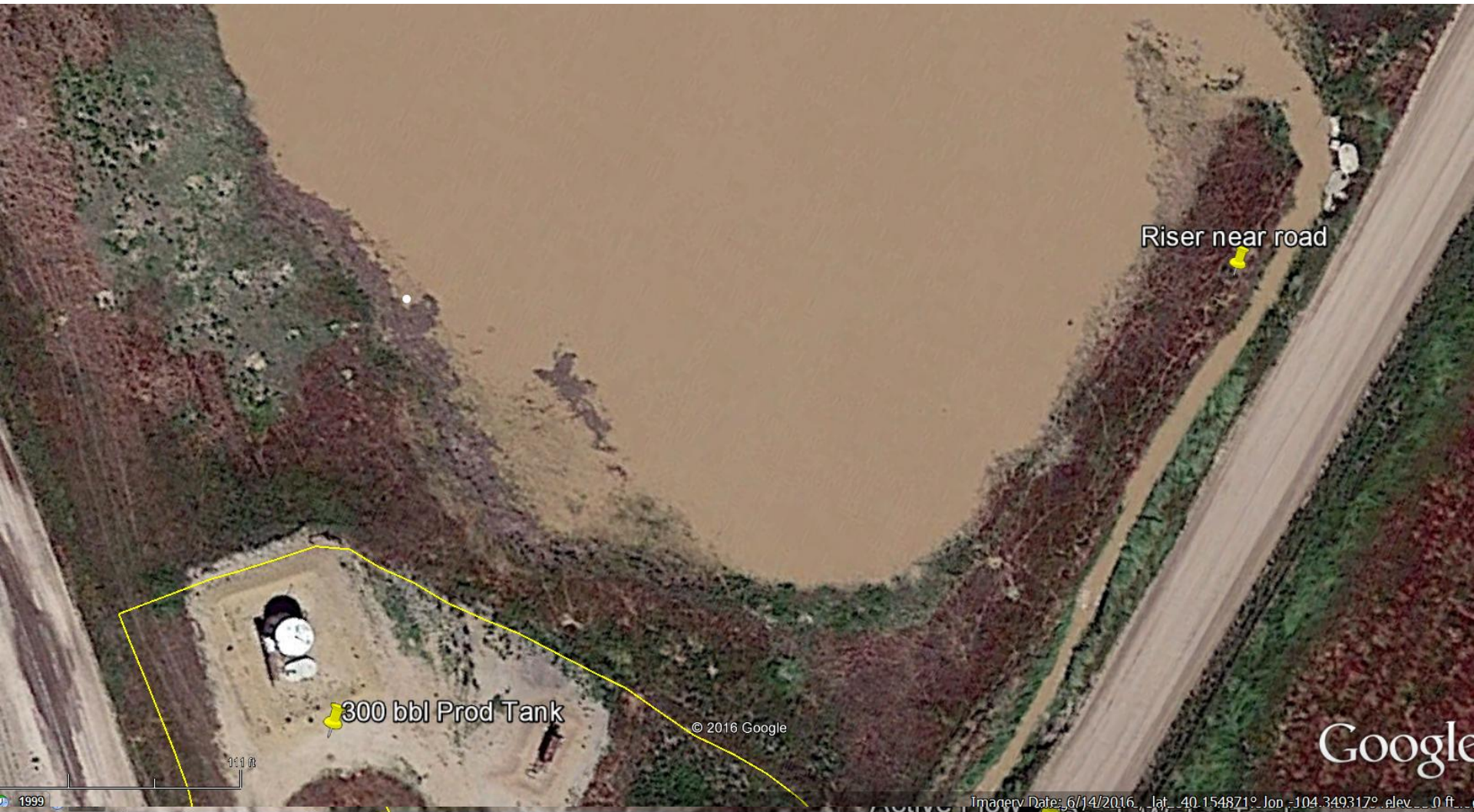
Photo 25: Aerial image. Photo shows location of a riser found near road, to the northeast of the location.
