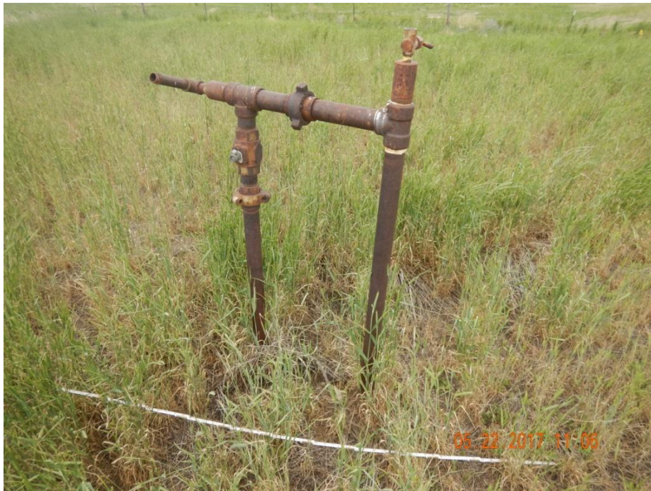
Photo 8: Photo of “~3 inch x2, connected at top”
