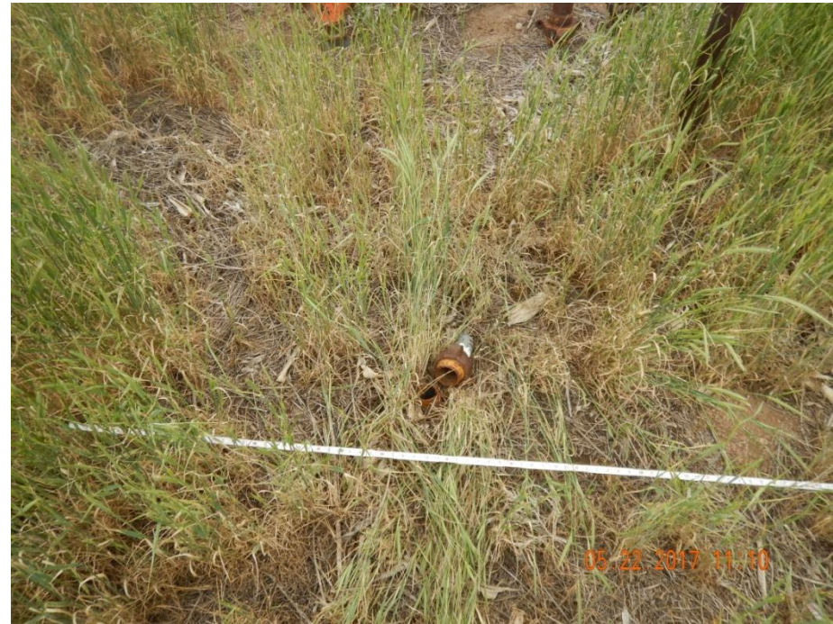
Photo 24: Photo of “~4 inch multi line w/ ~4 inch risers x2”
