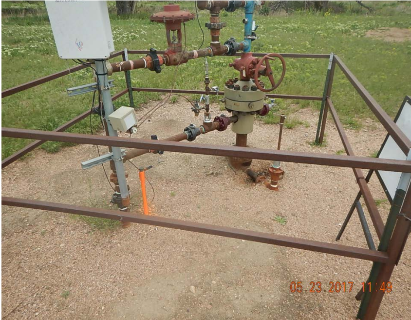
Photo 3: Risers at wellhead. Unused line marked for removal.
