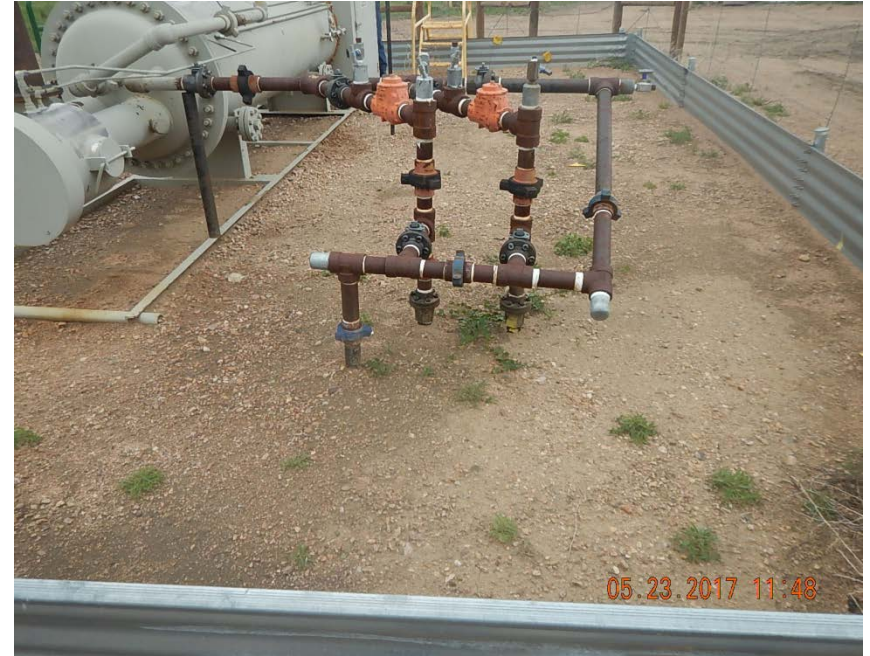
Photo 6: Risers at separator
