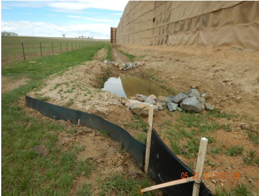
Photo 3. Photo taken from the western sediment trap, facing North. Sediment trap appears to be properly functioning. The Operator did not pump or direct stormwater from the location to this sediment trap.
