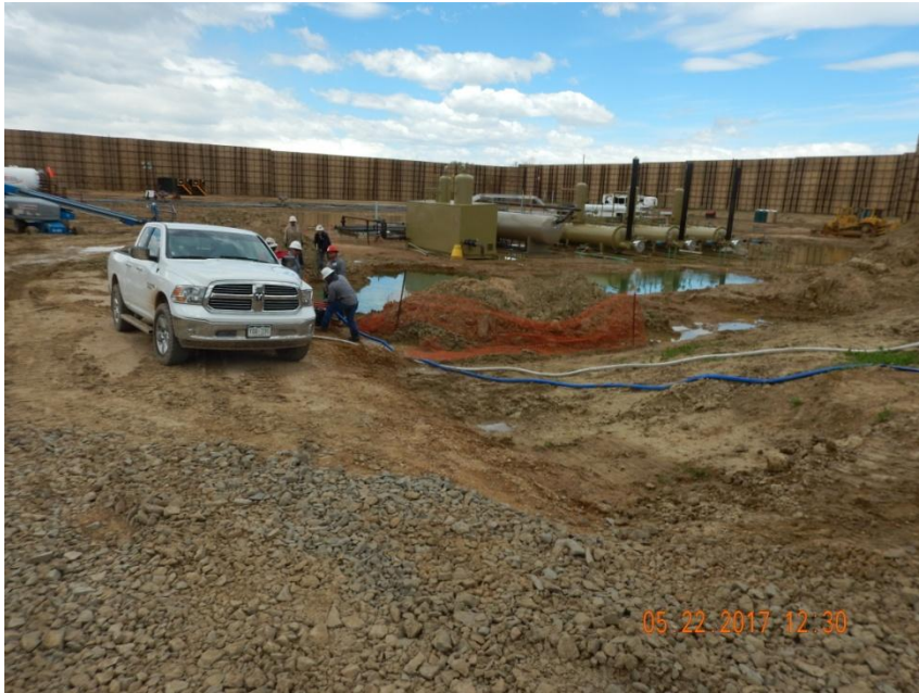
Photo 1. Photo taken from the entrance of the location, facing West. Photo illustrates the Operator pumping standing stormwater from location into the perimeter ditch BMP.
