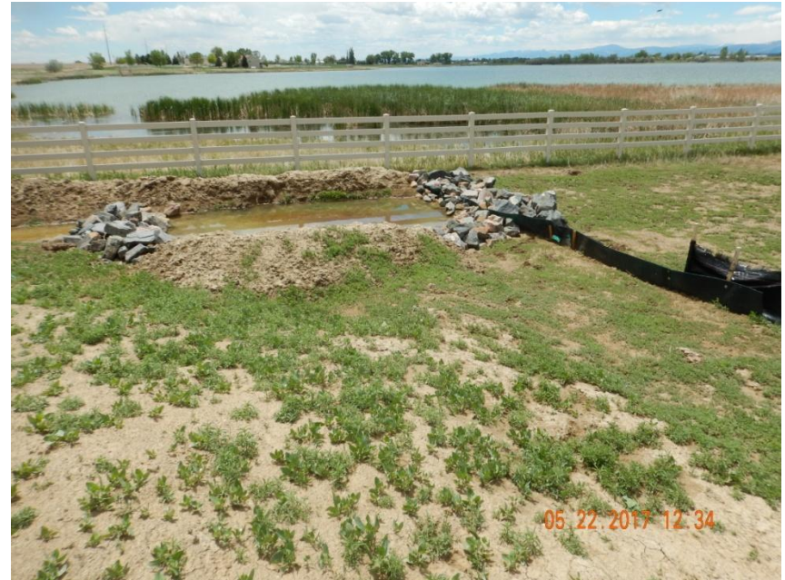
Photo 4. Photo taken from the southwestern sediment trap, facing South prior to the pumped stormwater from the location reaching the sediment trap. Sediment trap appears to be properly functioning at this time prior to pumping.
