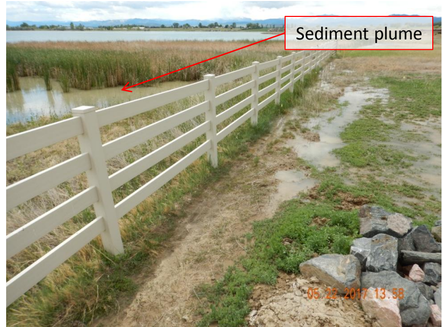
Photo 8. Photo taken from the southwest sediment trap, facing West. Photo illustrates pumped sediment laden stormwater from the location being discharged from location and areas west of the sediment trap that are contributing to additional sediment discharge into Newell Lake, ~20'-30' from the sediment trap. Photo also illustrates the sediment plume from sediment laden stormwater discharge flows from the location.
