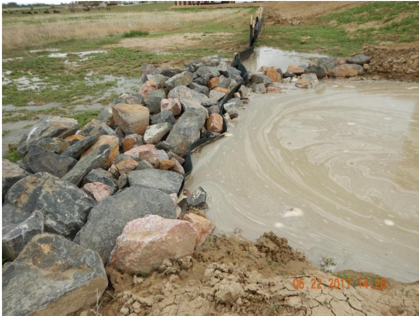
Photo 7. Photo taken from the southwest sediment trap, facing North. Photo illustrates pumped sediment laden stormwater from the location flowing through the sediment trap outfall at an accelerated rate that is not allowing sediment to drop out prior to being discharged from location, even with the S-Fence BMP.
