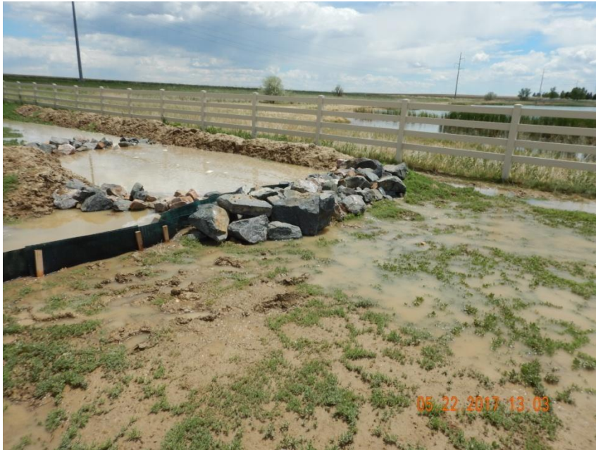
Photo 5. Photo taken from the southwest sediment trap, facing Southeast along the outfall area. Sediment laden stormwater is flowing through the sediment trap at an accelerated rate that is not allowing sediment to drop out prior to being discharged from location. S-Fence BMP does not appear to be an adequate BMP. In addition, discharged flows from the sediment trap are eroding the surface owners property off of the location west of the sediment trap which is contributing to additional sediment discharge into Newell Lake.
