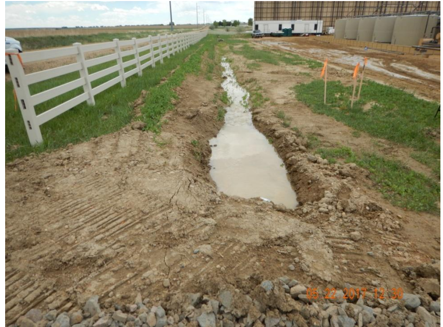
Photo 2. Photo taken from the entrance of the location, facing South along the perimeter ditch BMP. Photo illustrates standing stormwater from location being pumped into the perimeter ditch BMP.
